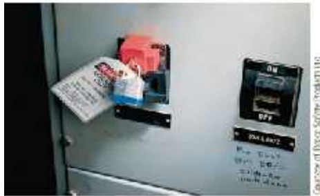
Figure2.2 Main Switch/MCB Isolation, Lock and Tag
