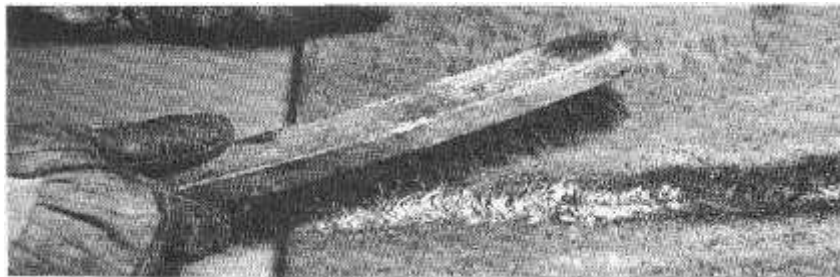
Figure 7 After chipping, brush the weld with a wire brush
