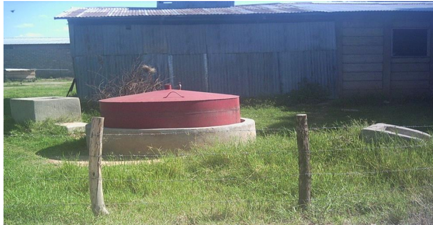
Picture (2): Floating Biogas Plant
