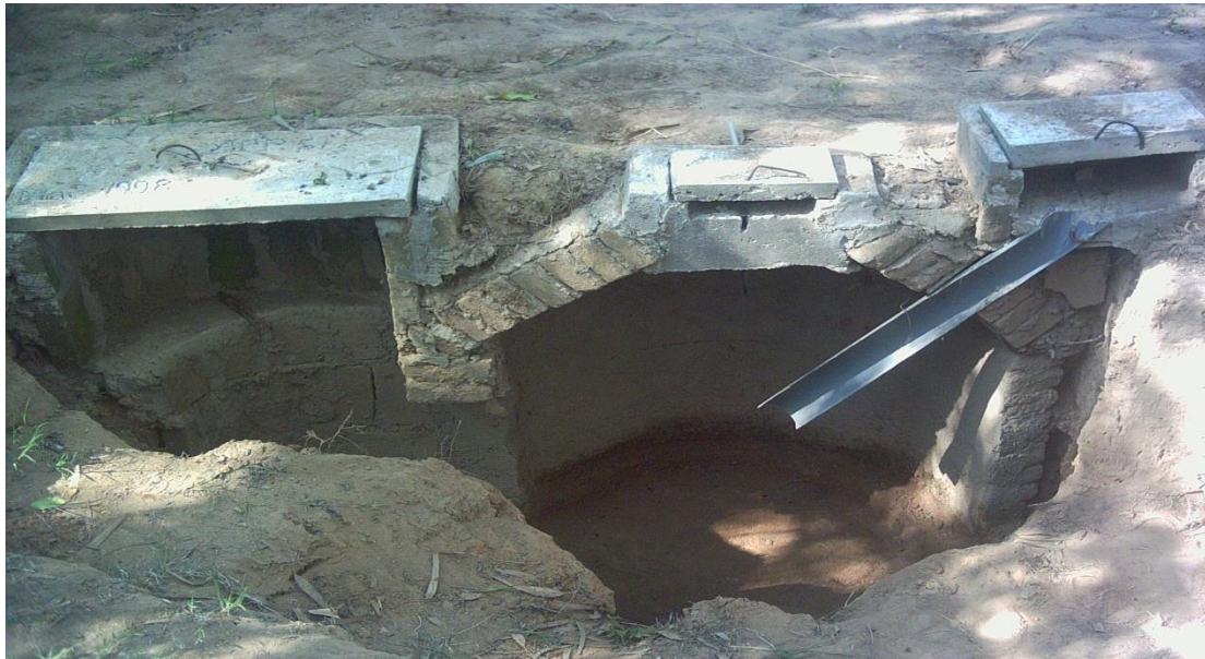
Picture(1): Fixed Dome Biogas Plant.
