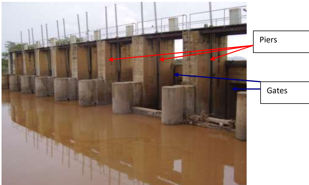
Fig: A barrage across a river
