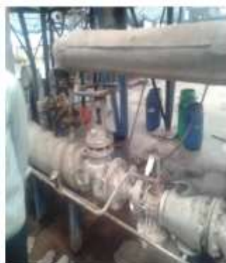
Opening Steam, water and air valve
