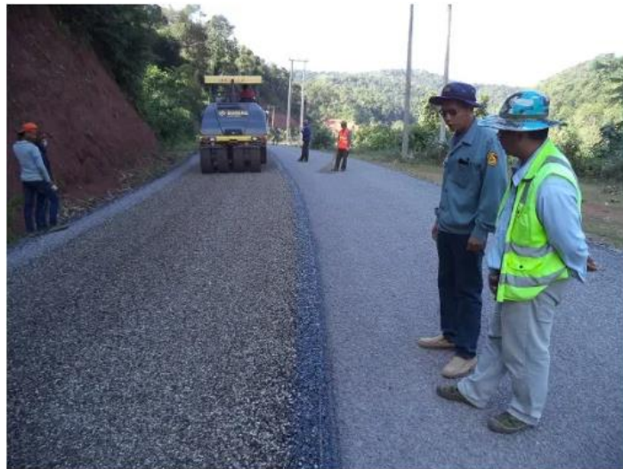
Figure 1-1 Asphalt Surface Treatment
