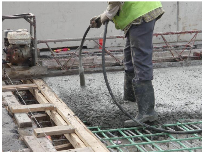
Figure 2. 6 Vibrating concrete
