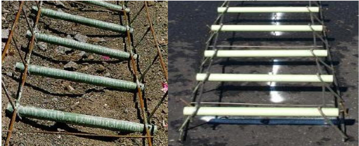
Fig.1. 26: Dowel bars
