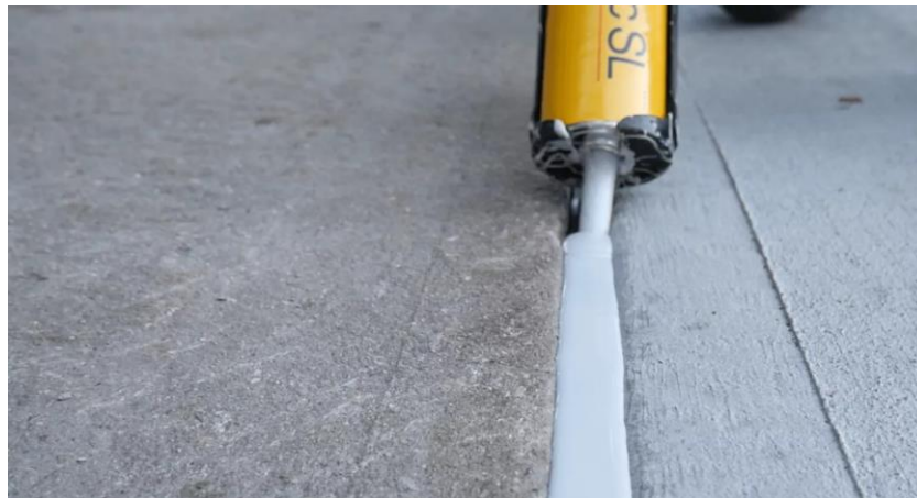
Fig1.34 Expansion joint sealant in concrete pavement
