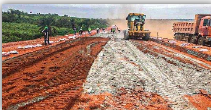
Fig 1-9 A truck applies cement stabilizers to a roadway
