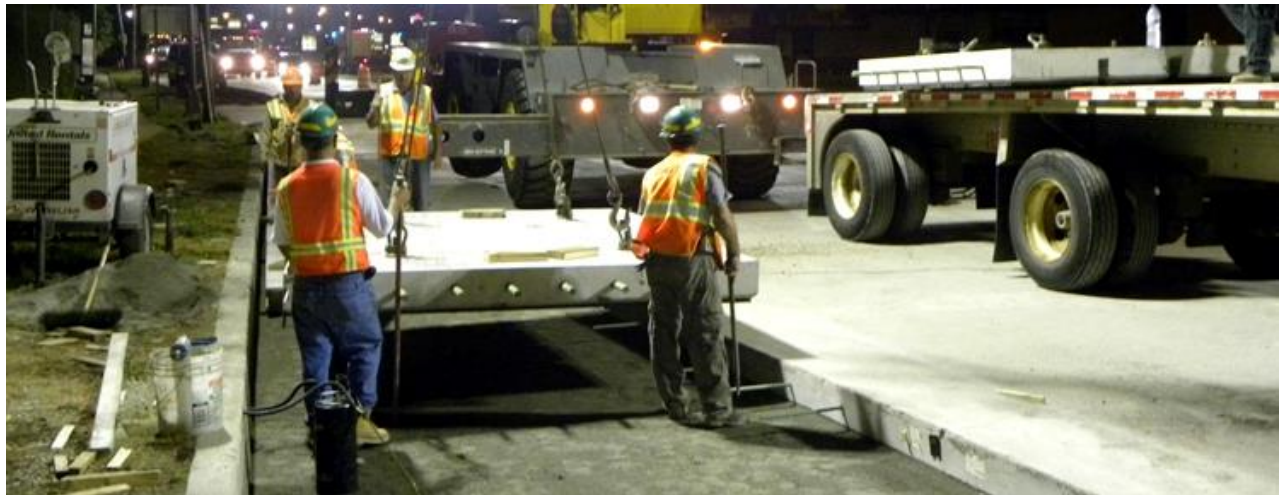
Fig1.17 Pre stressed concrete pavement (PCP)
