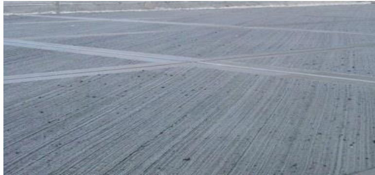
Fig 1.49: Broom Finished Concrete.
