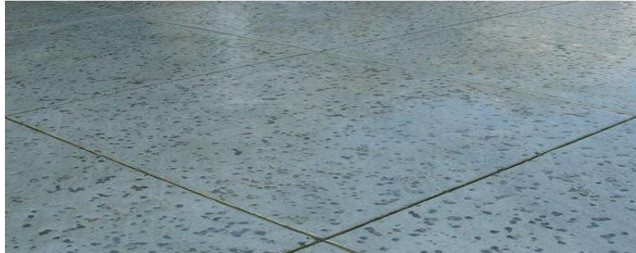
Fig 1.51: Salt Finished Concrete.
