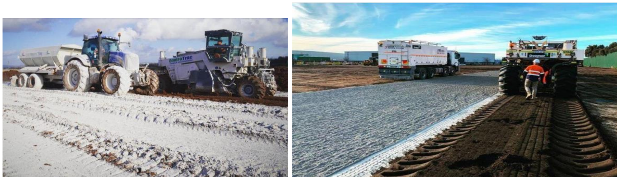
Fig 1-10 A truck applies chemical stabilizers to a roadway for dust suppression
