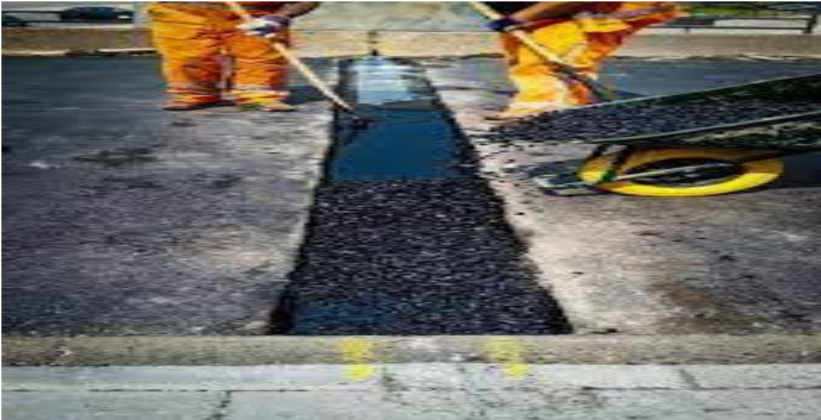
Figure 3-4 Joint Repair
