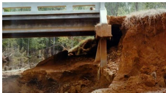
Fig 4.2 Erosion in bridge construction
