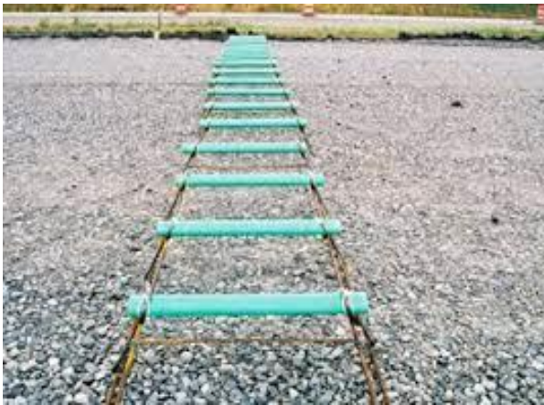
Fig1.43 Epoxy-coated dowel bars.
