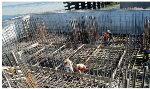
Fig 3.4 Cut and bent tied/fixed reinforcing
