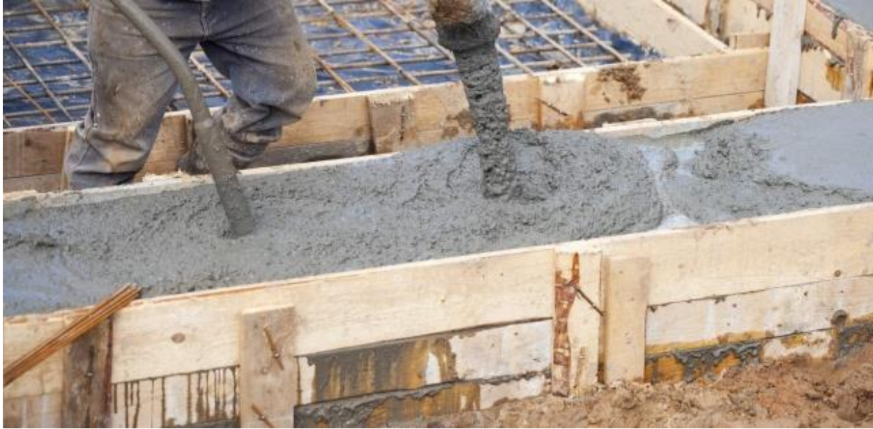
Figure 2. 4 Concrete placing
