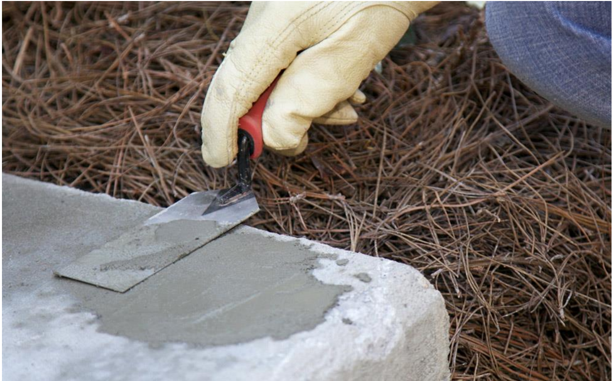
Figure 4. 6 Finishing Concrete
