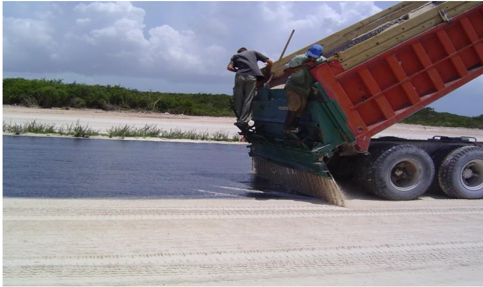
Figure 1-3 Sand Seal
