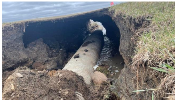
Fig 5.7 Repairing inlet and outlet
