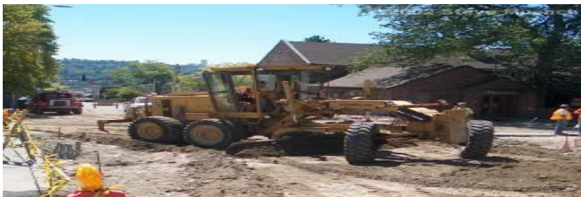
Figure 1.4: A grader preparing the sub grade on a project
