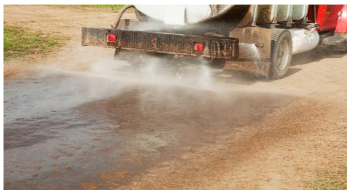
Fig 1-12 A truck applies chemical stabilizers to a roadway for dust suppression
