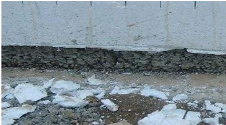
Fig 1.47 Concrete Segregation
