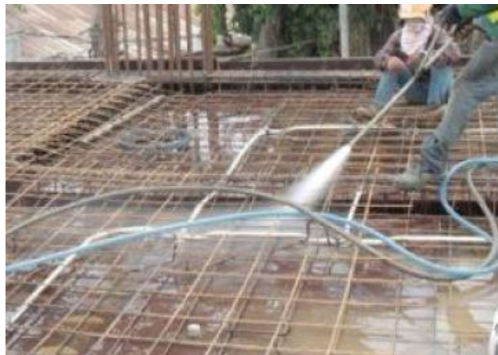
Fig1.45 formwork water tight
