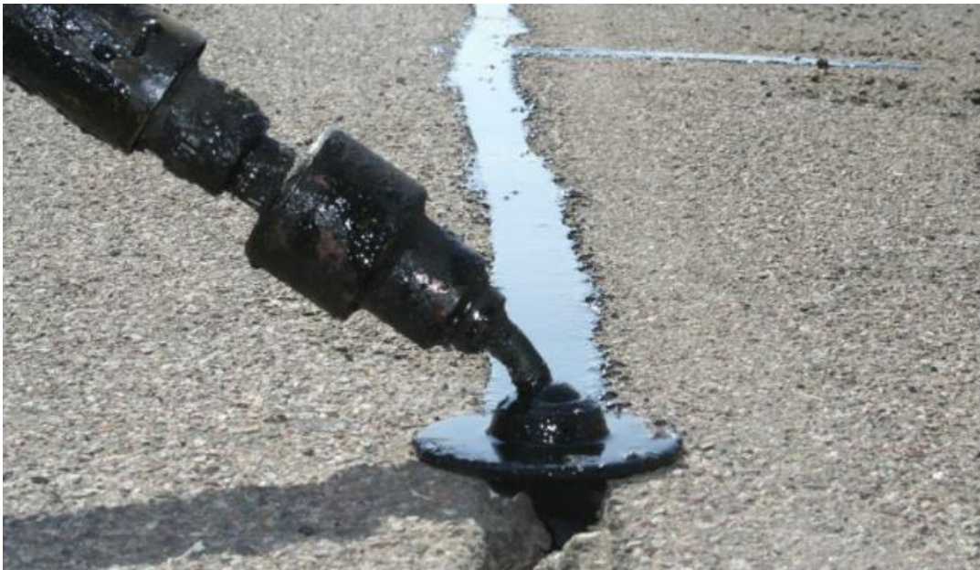
Figure 3-3 Crack Sealing
