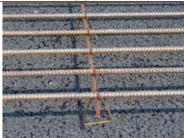
fig1.16 Transverse Bar Assembly
