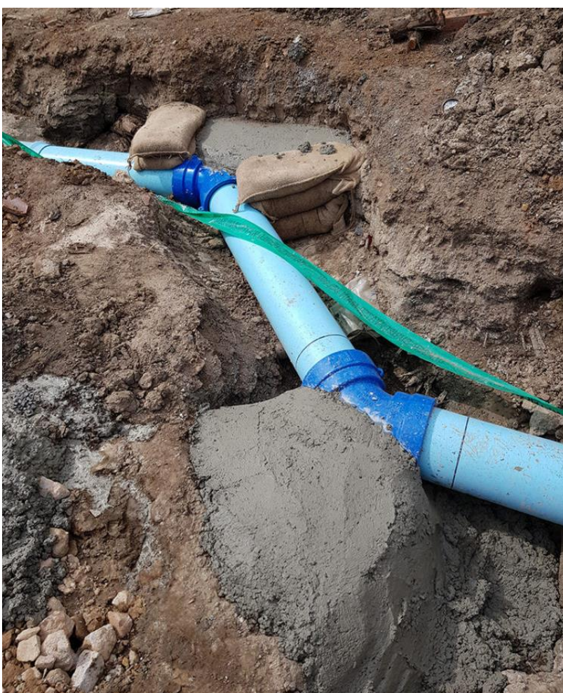
Figure 3. 30 Thrust blocks
