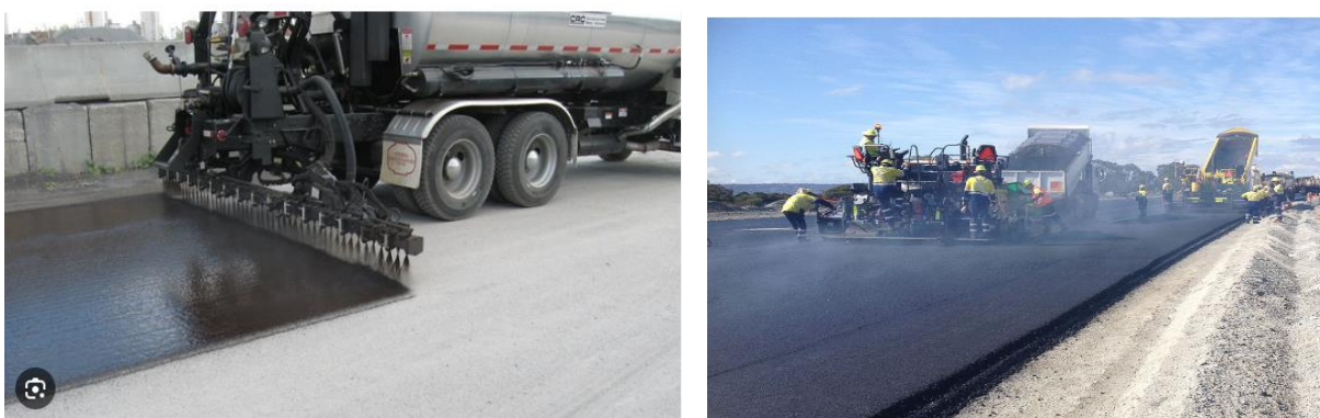
Fig 1-11A truck applies Bitumen stabilizers to a roadway
