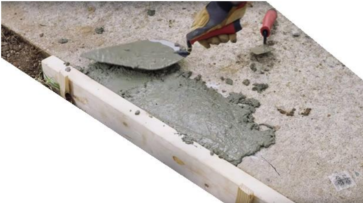
Figure 4. 5 Setting up formwork use to replace removing section
