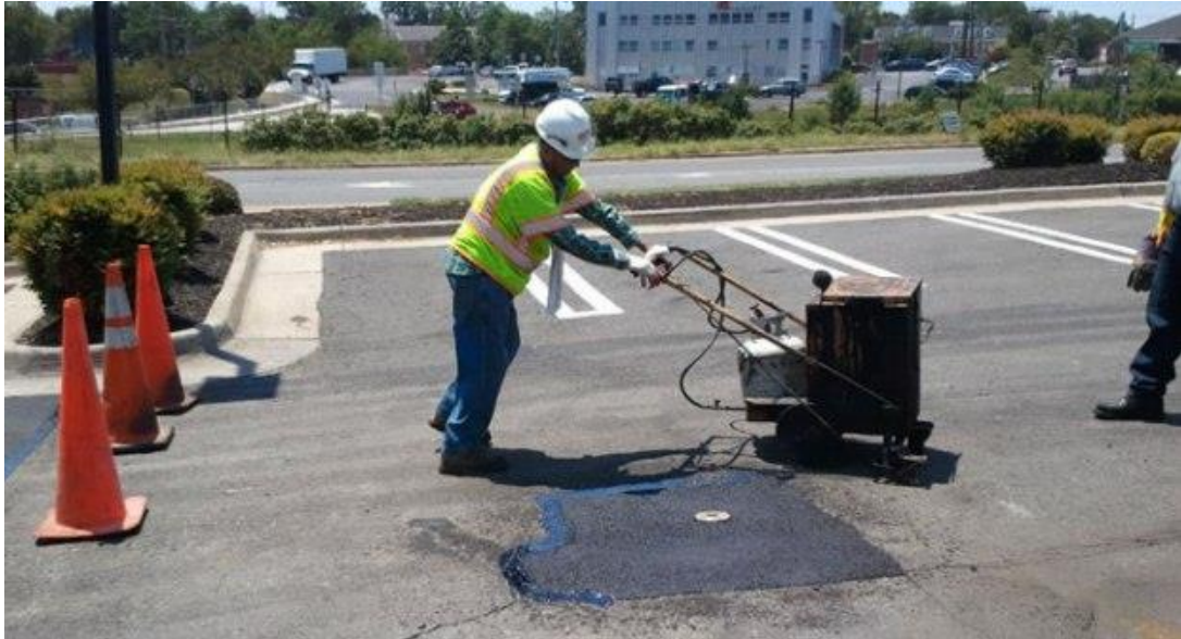
Figure 2-8 Patching and Pothole Repair
