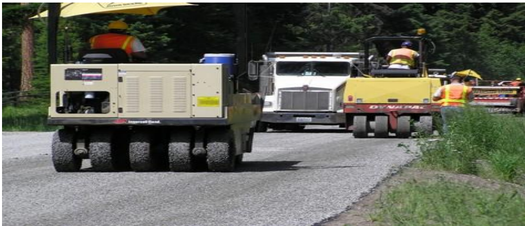
Figure 1.12: A pneumatic tire roller compacting chip seal.
