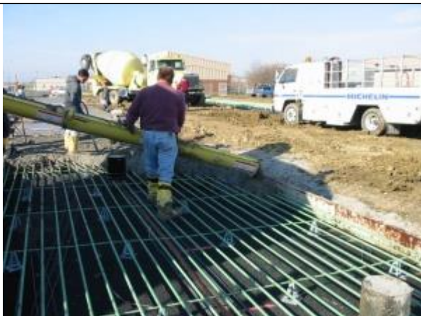
fig 1.15 CRCP Hand Placement
