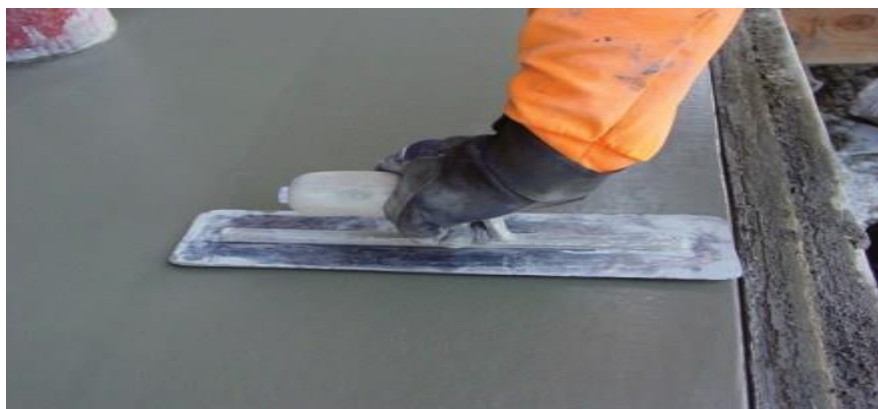
Fig 1:48 Trowel Finished Concrete.
