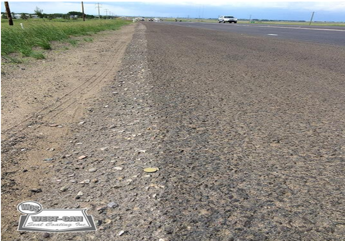
Figure 2-7road surface for sand seal application
