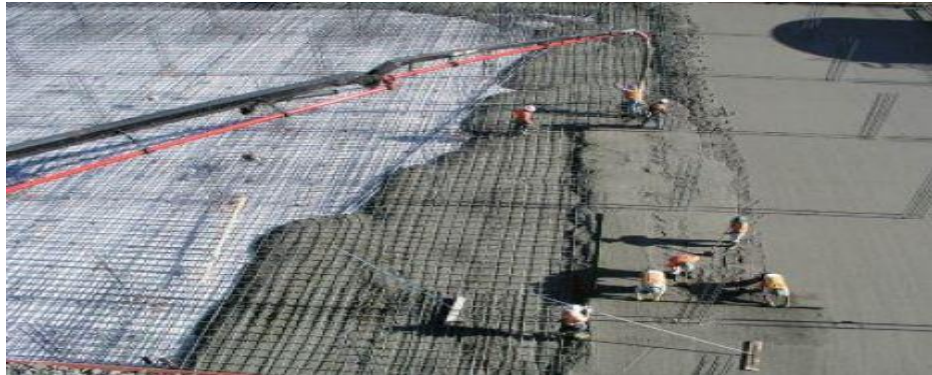
Fig 1.46 Concrete Placement Layers
