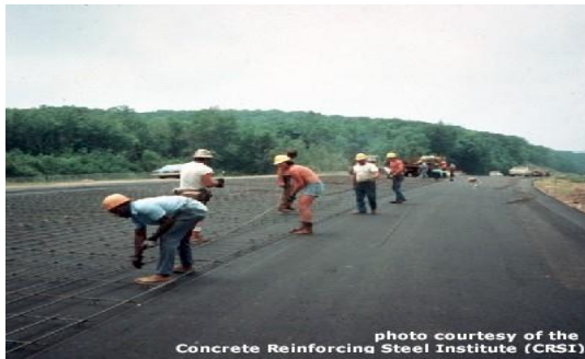
Figure1.25. Tie Bar placement
