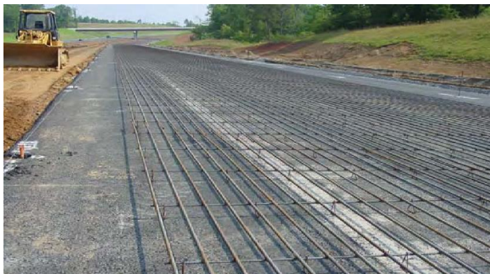
Fig1.3 Steel reinforcement used in rigid pavement
