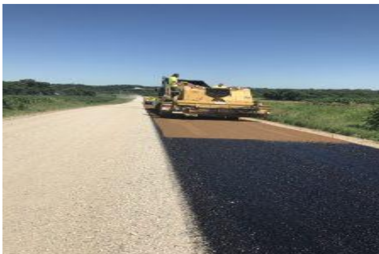
Figure 1-2 Otta Seal
