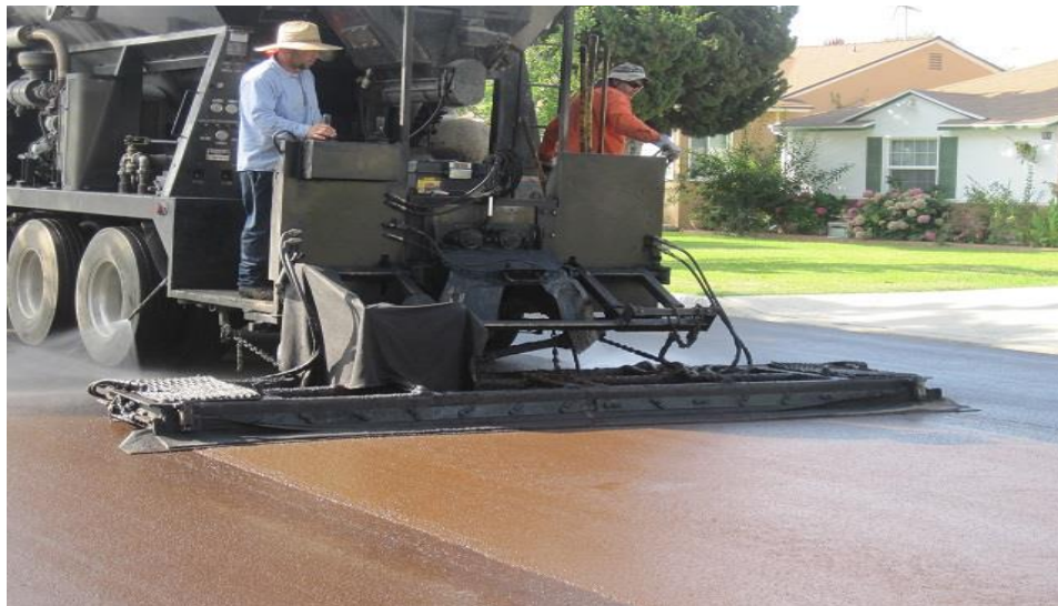
Figure 1-4 Slurry Seal
