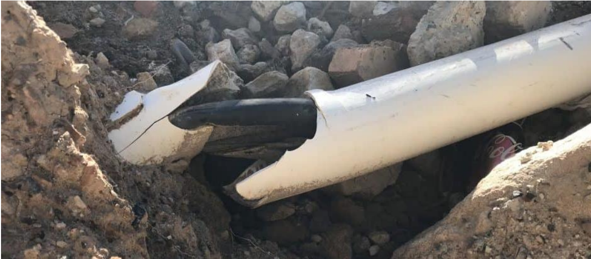
Figure 2. 1 Accidental damage to underground services
