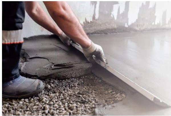
Fig 3.6 finishing the concrete
