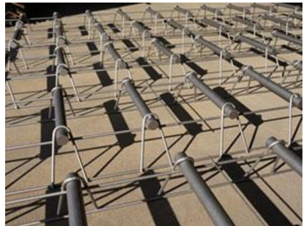
Fig1.41 Stainless steel dowel bars
