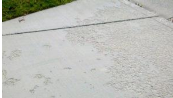
Figure 4. 2 Spalling
