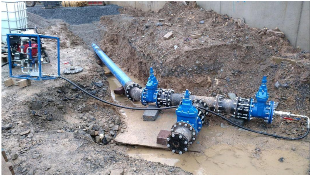
Figure 3. 15 Pressure testing
