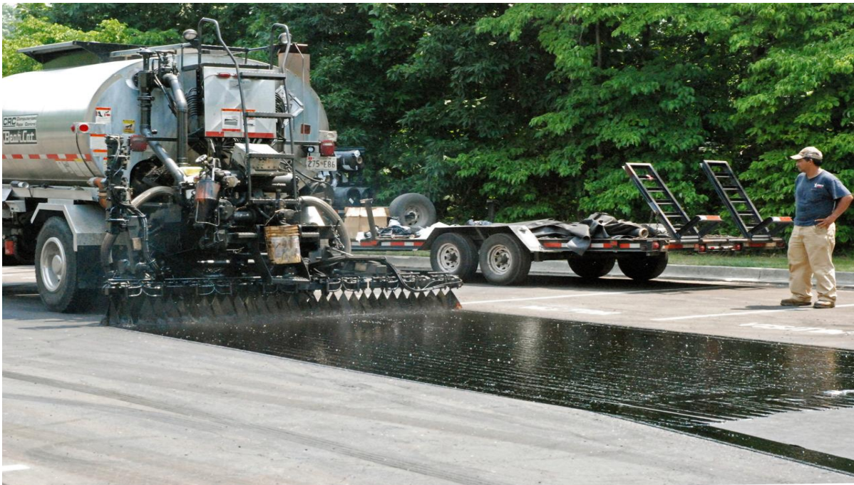
Figure 2-5 Road surface for asphalt surface treatment.
