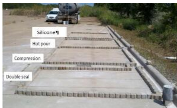
Fig1.5 Joint sealer used in rigid pavement
