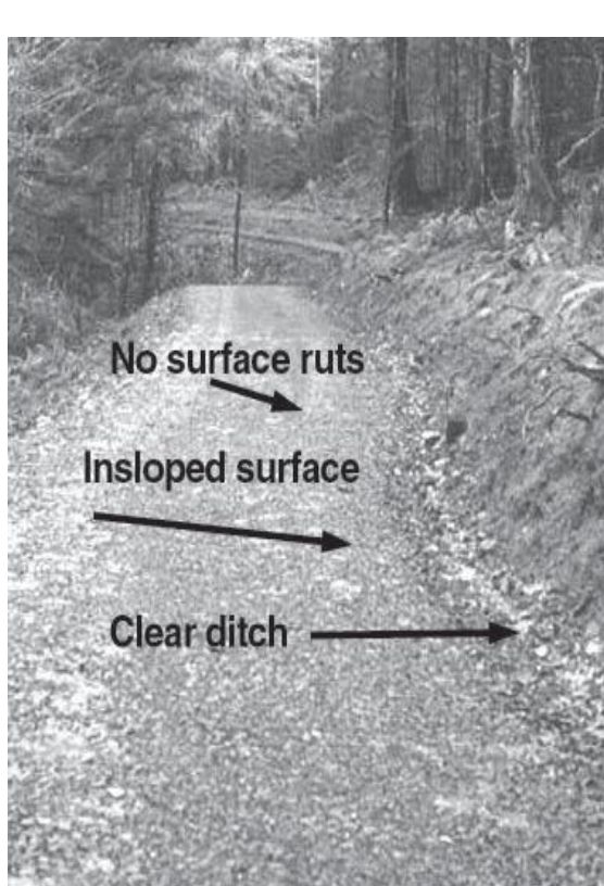
Fig.3.A well-maintained ditched road.
