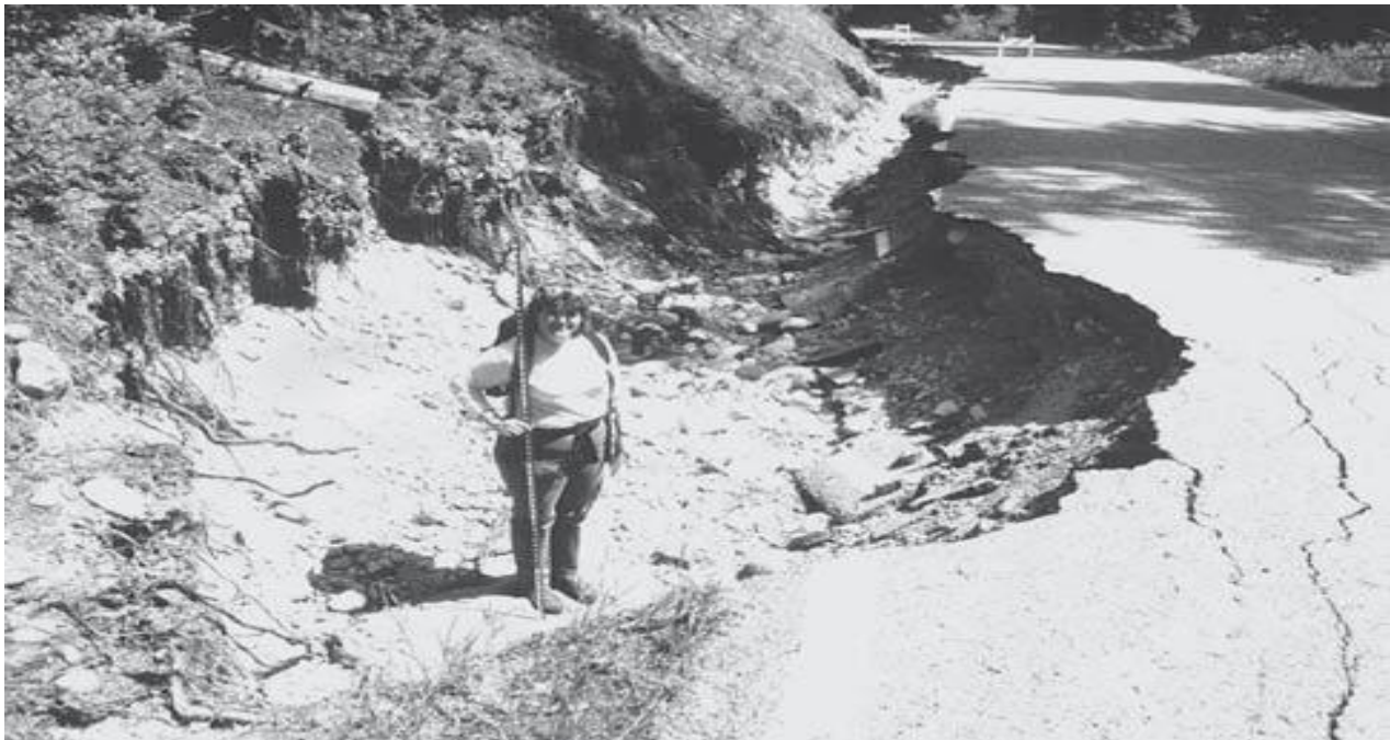
Fig.11. Significant ditch erosion
