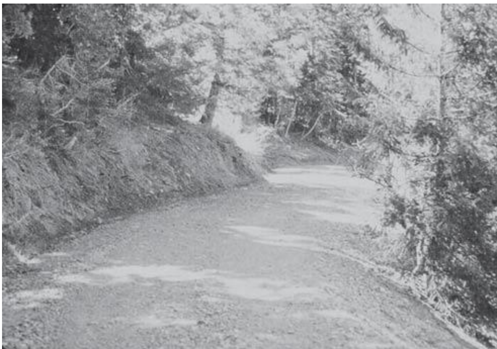
Figure 4-9. Road constructed with well-compacted and –drained subgrade
