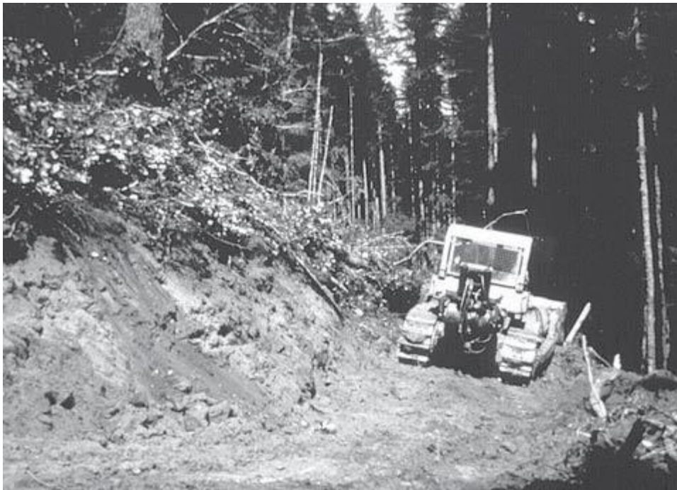
Figure 4-2. Tractor clearing and grubbing.
