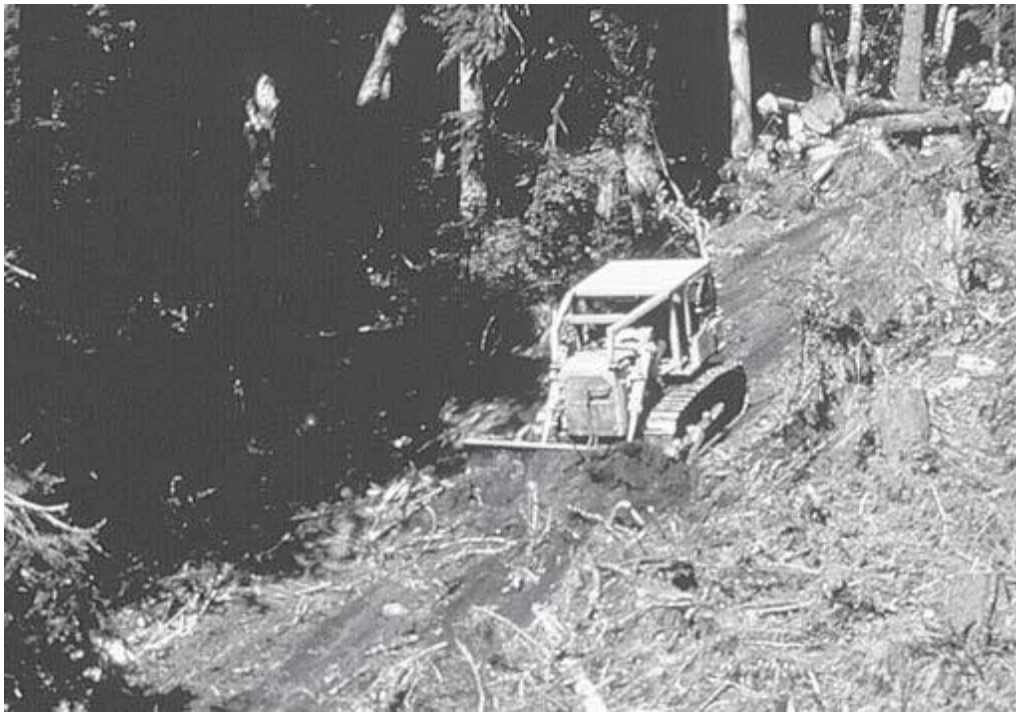
Figure 4-6. Tractor constructing road subgrade.
