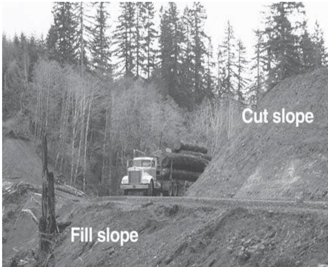
Figure 1-8. Example road cut and fill slope.
