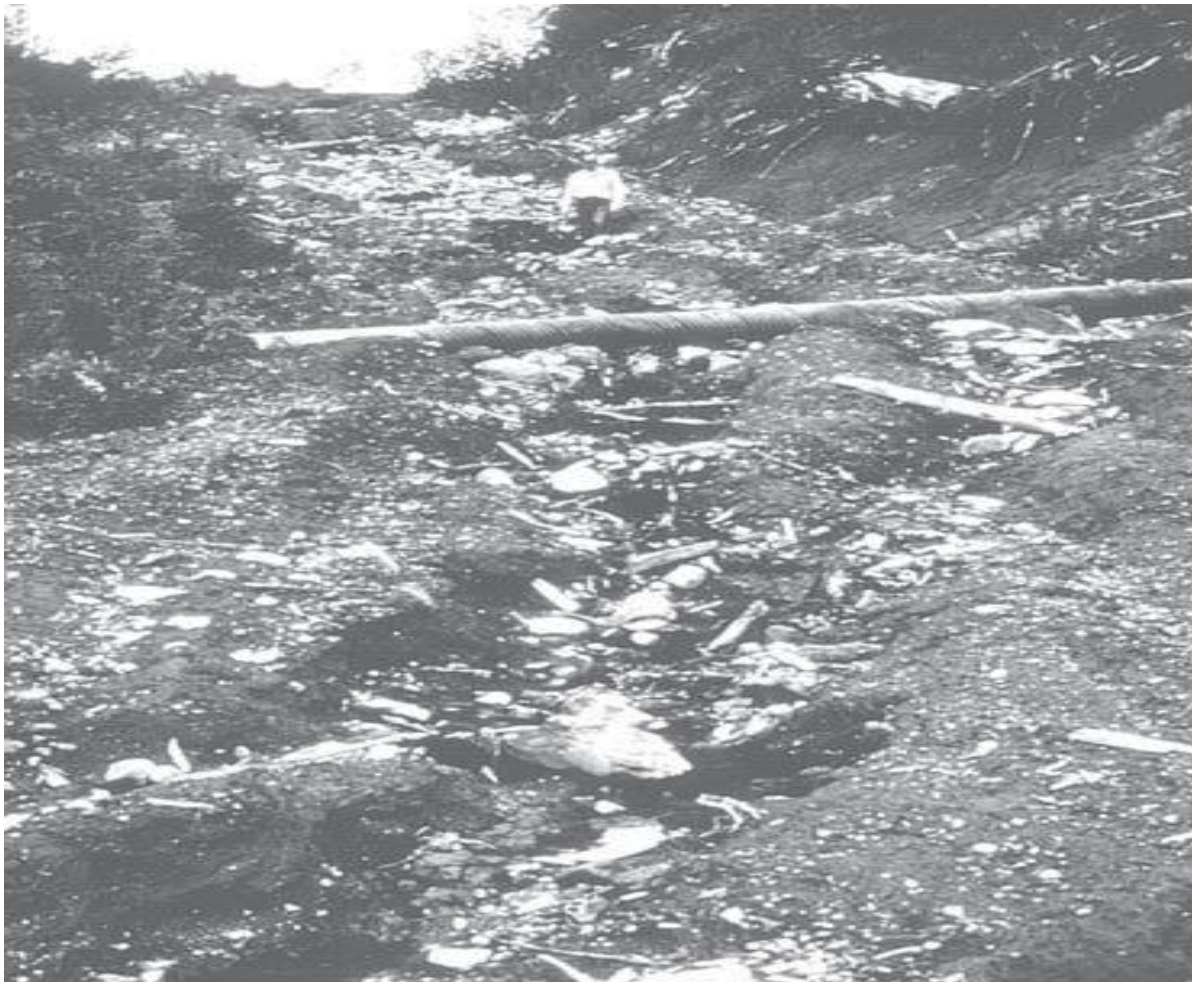
Fig.10.Catastrophic ditch and roadway erosion
