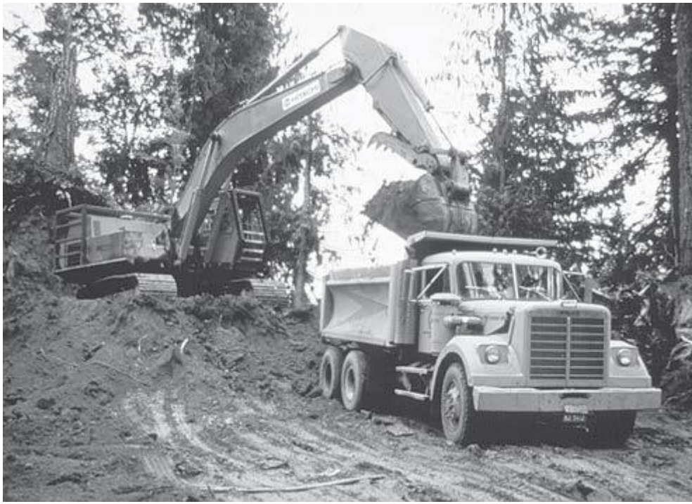
Figure 4-7. Hydraulic excavator excavating roadway material.
