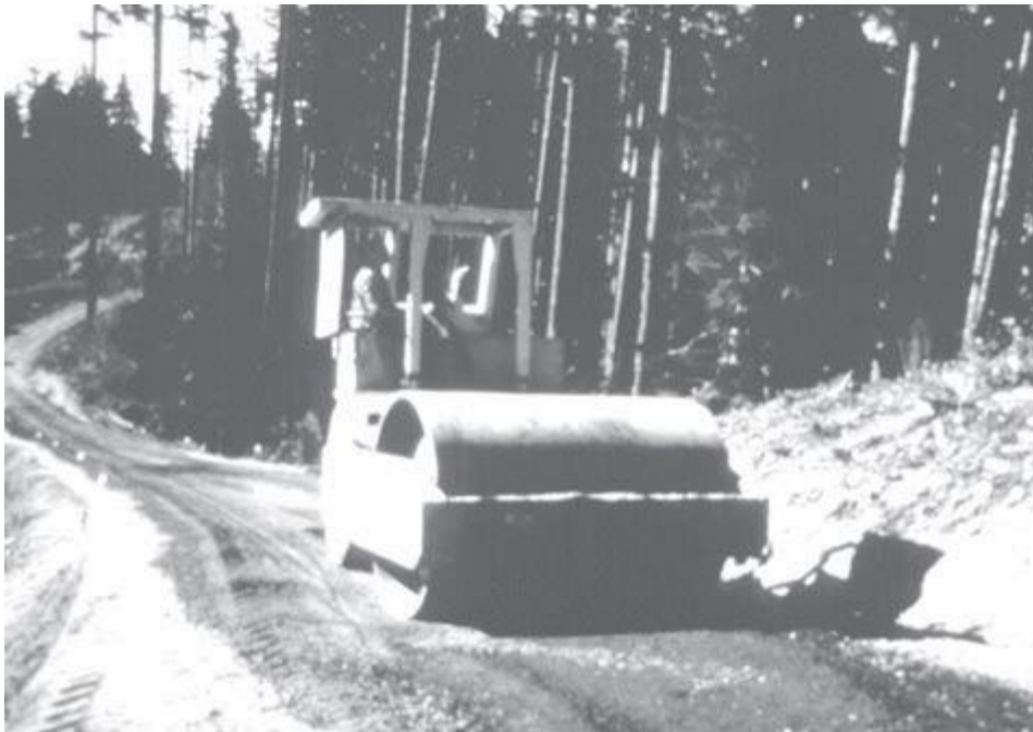
Figure 4-15. Smooth-wheel vibratory roller compacting surface rock
