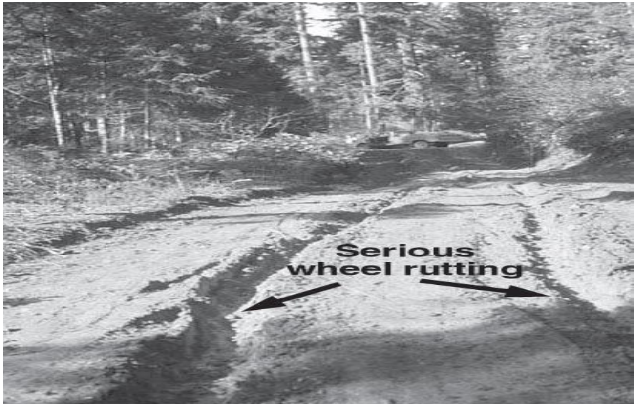
Figure .2 Excessive wheel rut damage to the road surface.
