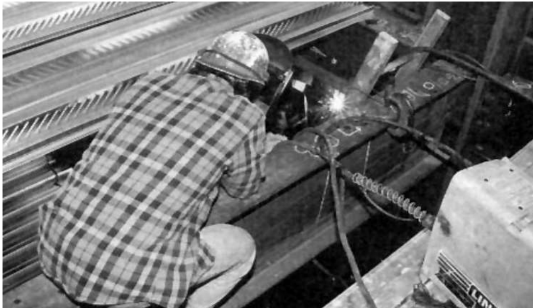
Figure 134: Effective visual inspection requires that the Inspector be present when welding is being performed.
