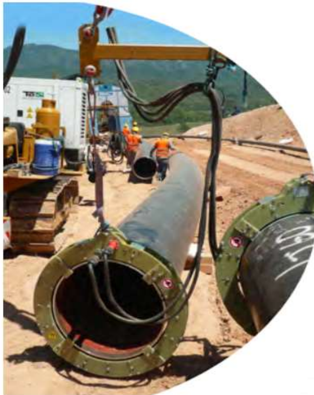
Figure 95: Heating Ring
