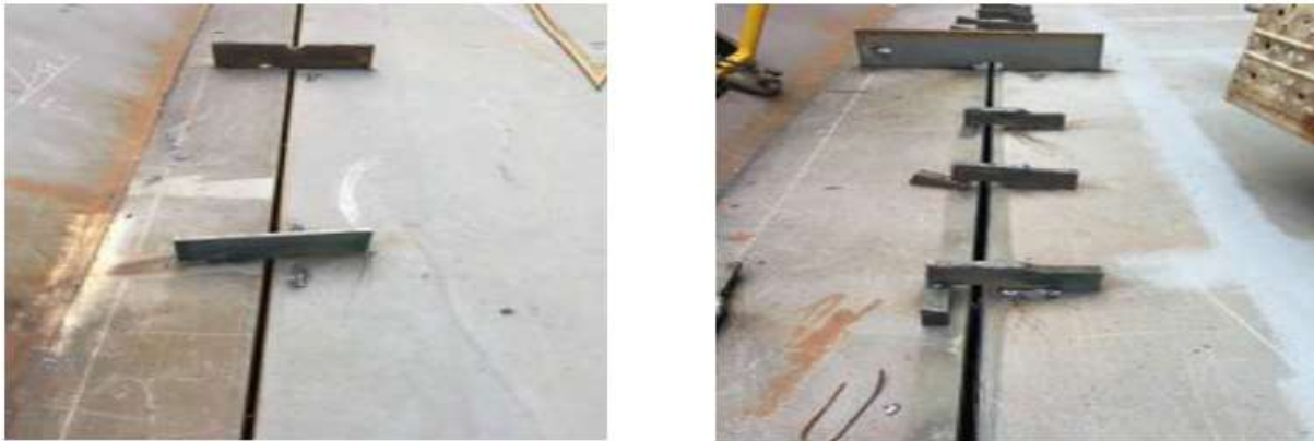
Figure 126: Fit-up with Welded Strong back and Wedges
