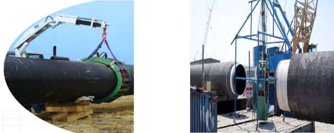
Figure 96: Clamp Coils - IWC
