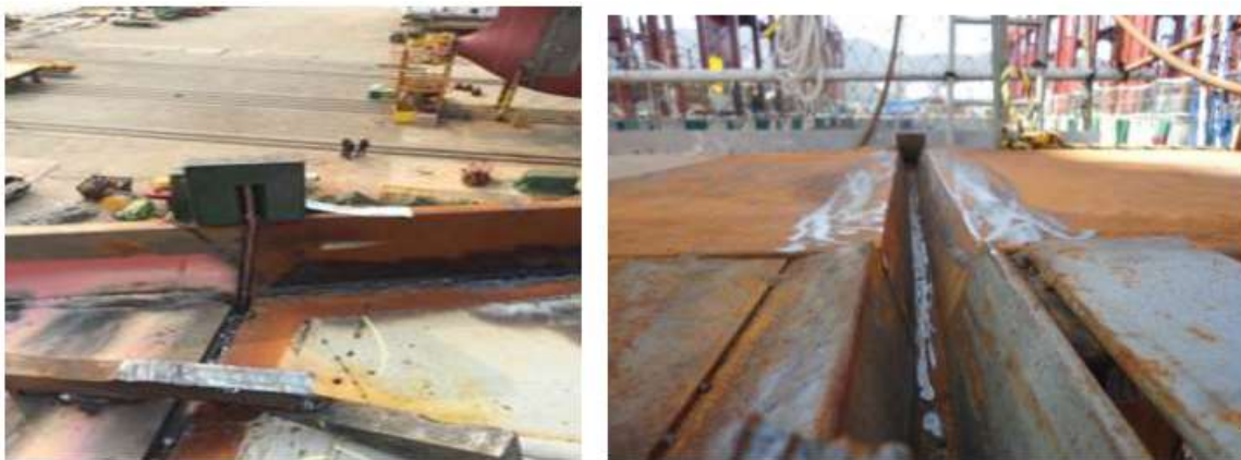
Figure 128: Correct Use of Tab Piece
