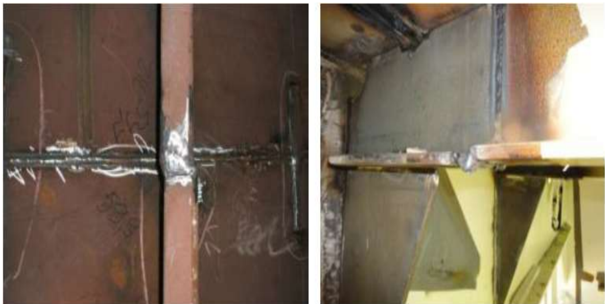
Figure 125: Poor Butt Joint Alignment and Poor Alignment of Stiffener Flange
