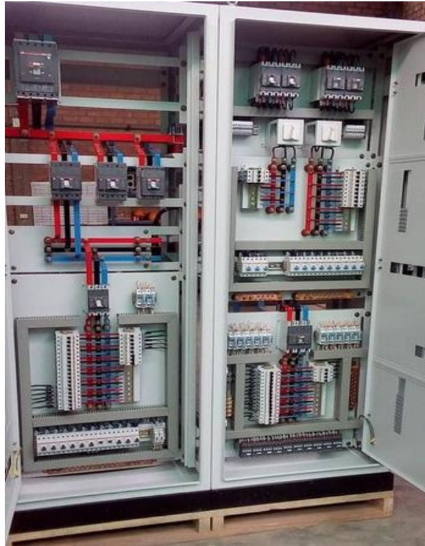
Fig 3.11. Fixing Wiring Accessories on Board
