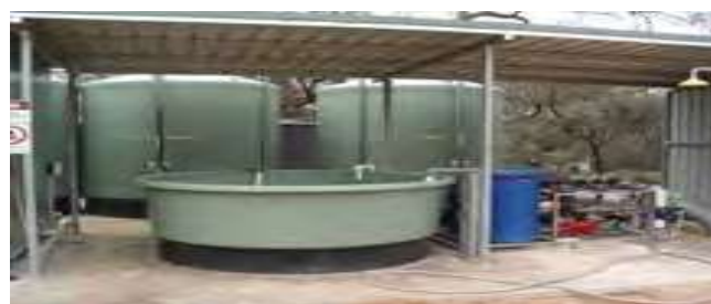
Figure 2.2. Fully automated twin multi-tank fertigation system.
