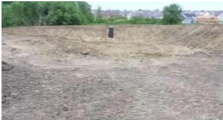
Figure 2.6. Sediment basin
