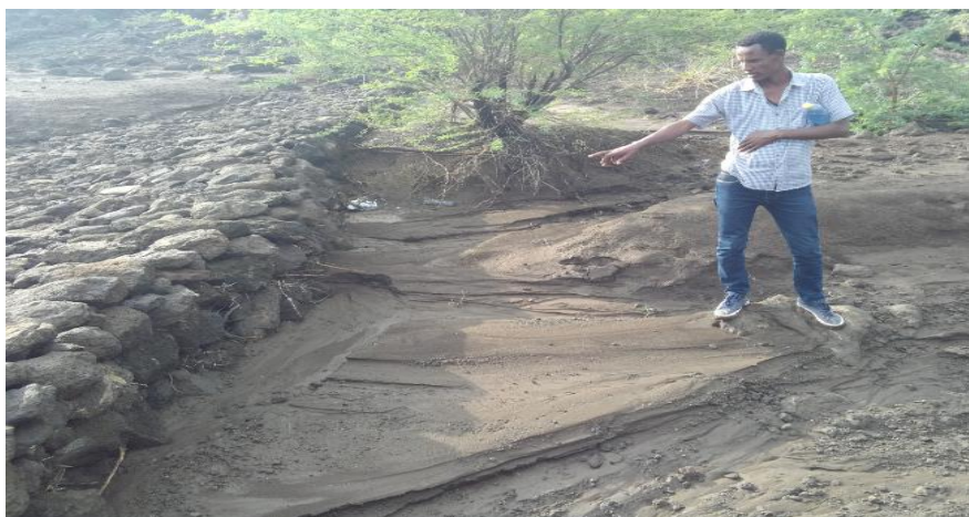
Figure 2.3. Sediment trap by DSM structure
