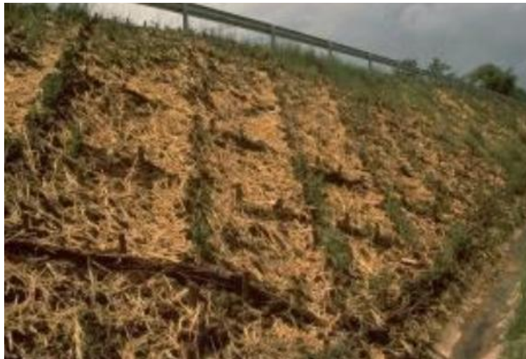
Figure 2.8. Mulching on soil
