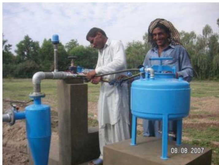
Figure 3.3 Head Unit Installation
