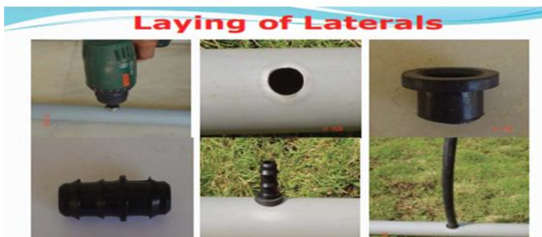
Figure 3.5 Laying Lateral Lines
