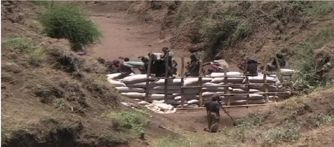
Figure 2.2.sandbag check dam
