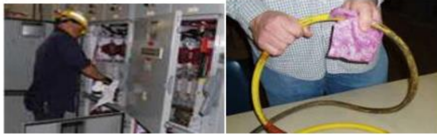
Figure 2.8 Clean out Look for tear/cut insulator
