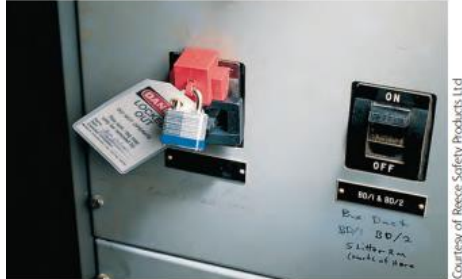
Figure 2.2 Main Switch/MCB Isolation, Lock and Tag
