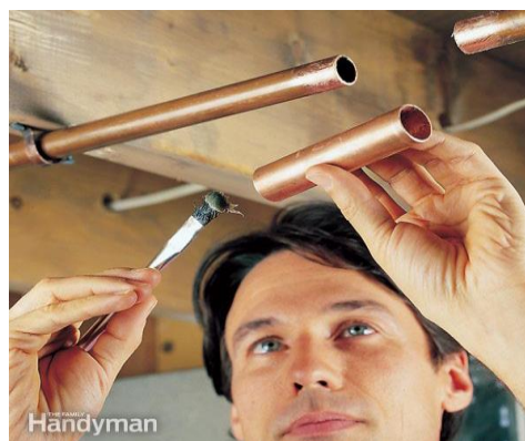
Figure 25 Cut out the damaged section
