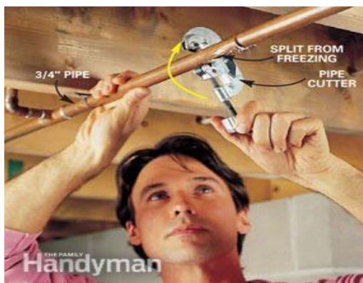
Figure 25 Cut out the damaged section
