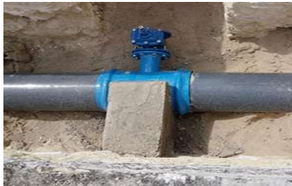
Figure 1.29.thrust block
