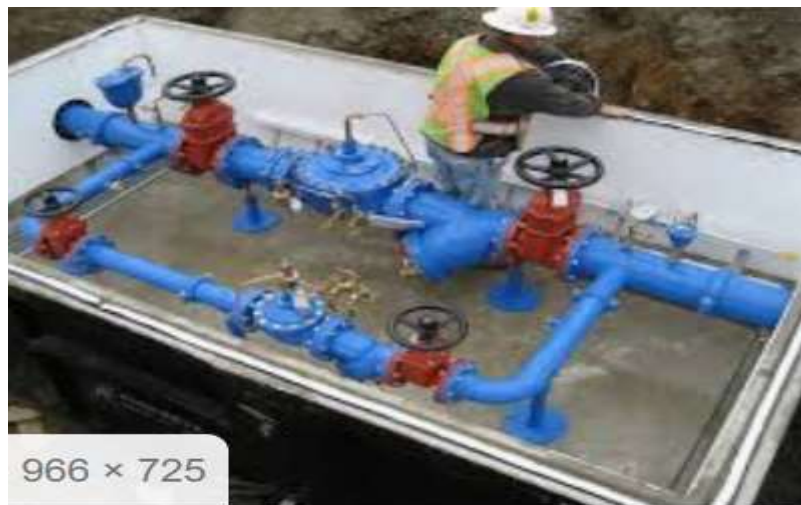
Figure 1.7. valve chamber
