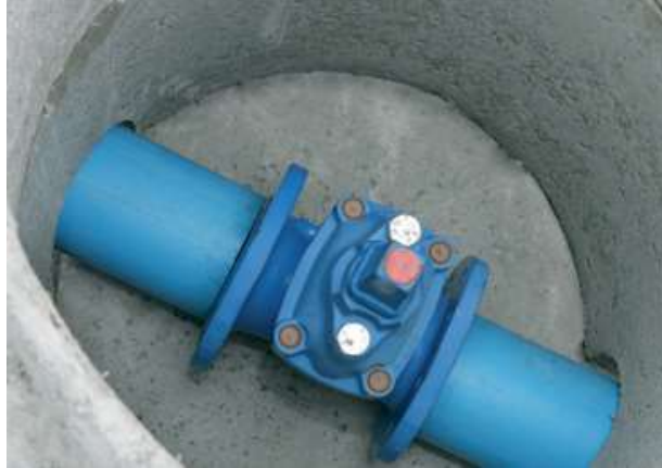
Figure 1.30. valve chamber
