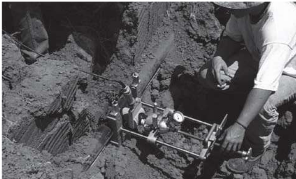
Figure 5.2 Saddle Fusion Repair
