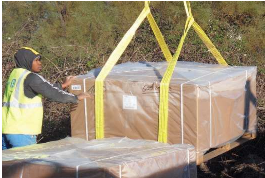
Figure 1.4: Transport of EF couplers, packed on individual pallets in horizontal position
