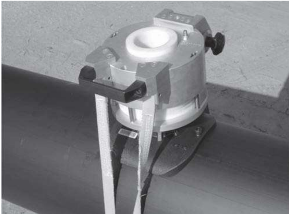
Figure 5.3 Electrofusion Patch Repair
