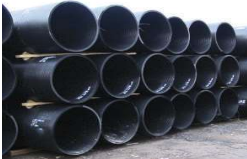
Figure 1.3 Example of good on-site PE Pipe Packing and Storage
