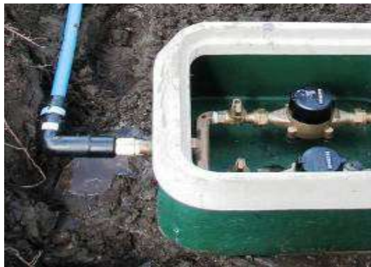
Figure 1.4a meter box mechanical coupling
