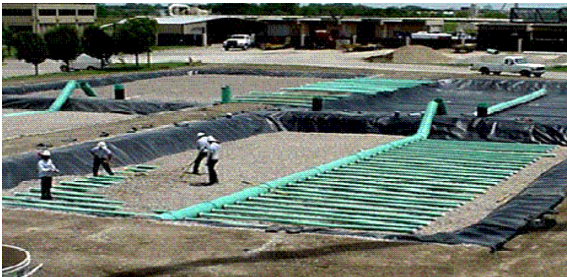
Figure 21: Photograph of four Biofilters being installed in Arlington, TX At Central Regional Wastewater System Plant
