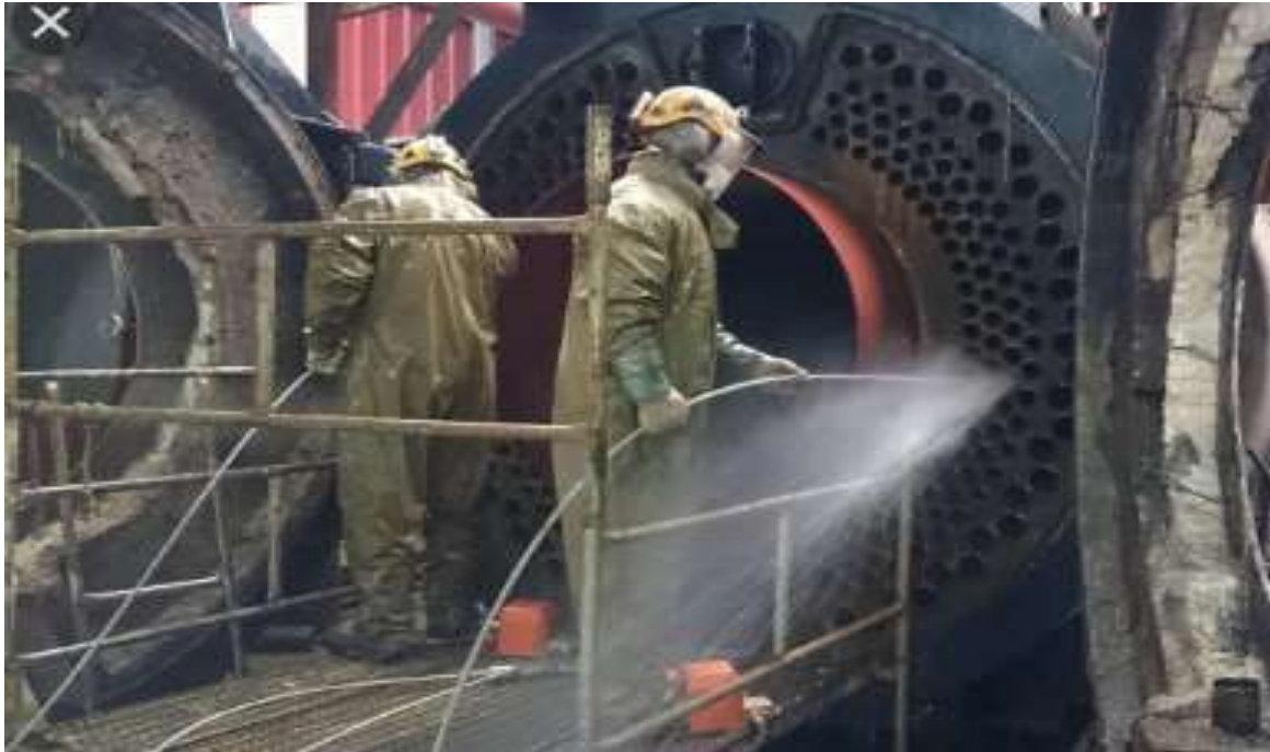
Fig 2 external cleaning of boiler
