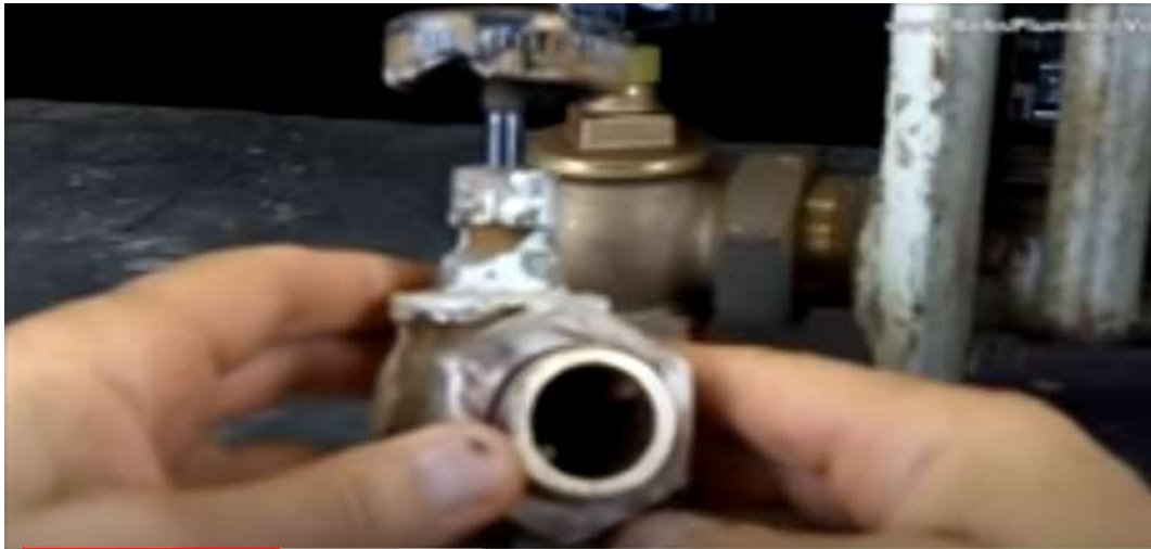
Fig 2 removing valve from boiler
