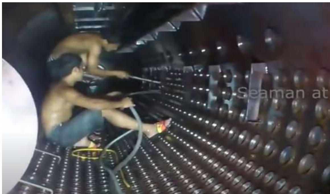
Fig 1 internal cleaning of boiler
