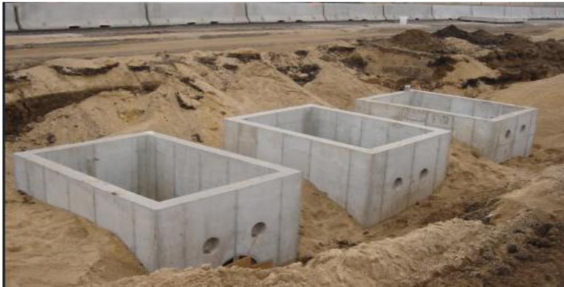
Figure 31: Prefabricated concrete drainage components in place
