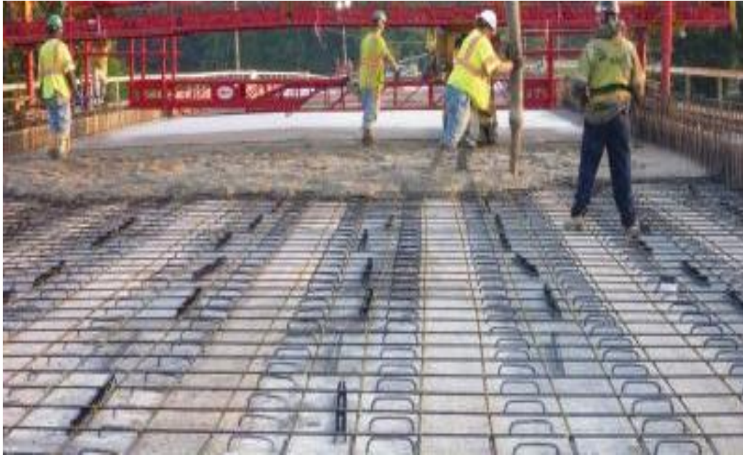
Figure 43: Placing of concrete within formwork
