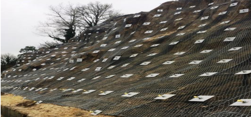
Figure 24: Soil nails
