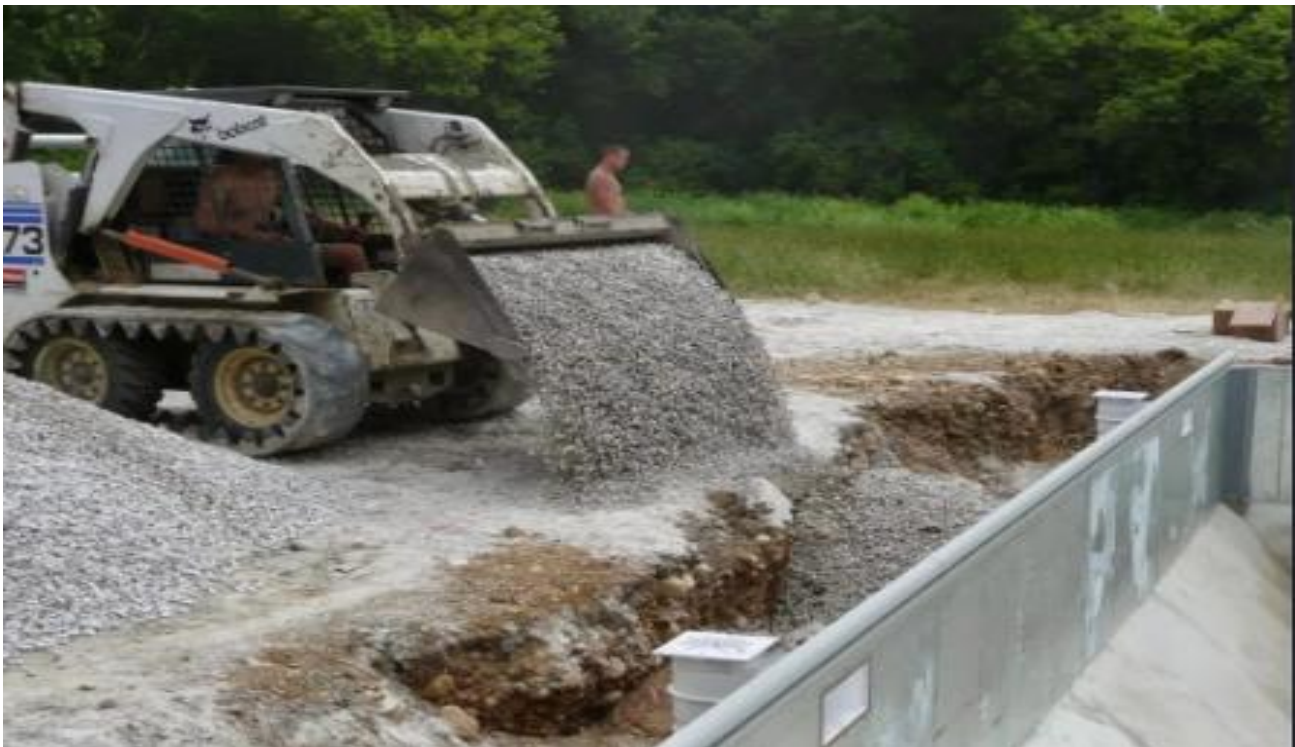
Figure 46: Backfilling
