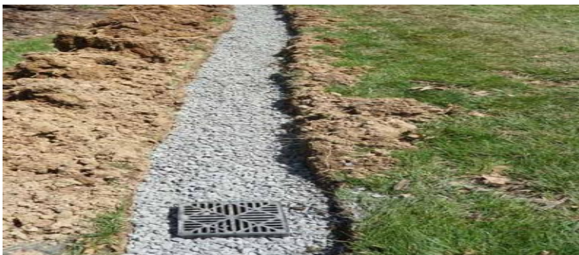
Figure23: French drains
