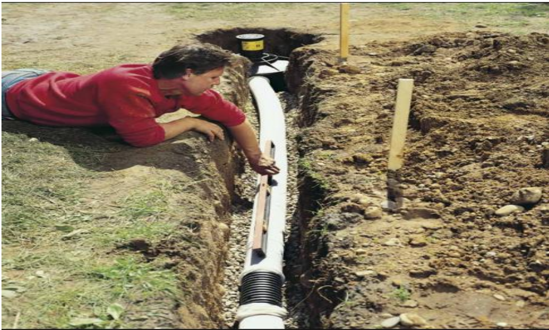
Figure 37: Checking the alignment of installed drainage pipe
