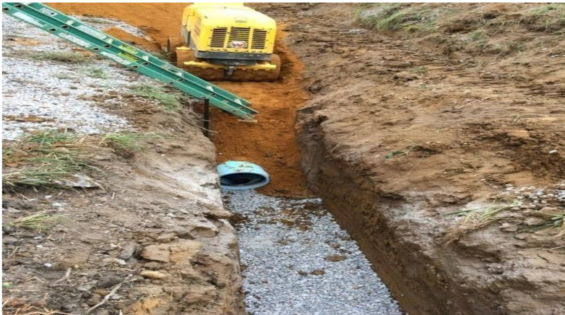
Figure 35: Final Backfilling and compaction
