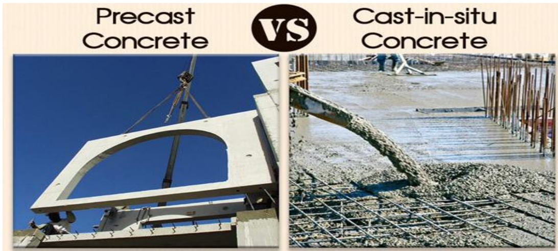
Figure 40: Differences between cast in situ and precast components.
