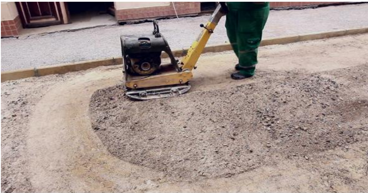
Figure 47: Compacting
