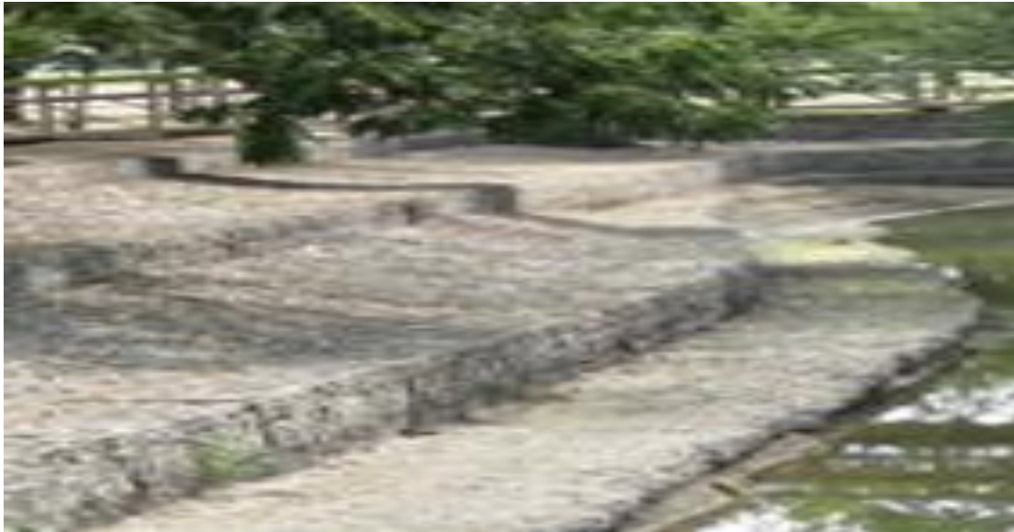
Figure 22: Gabion baskets
