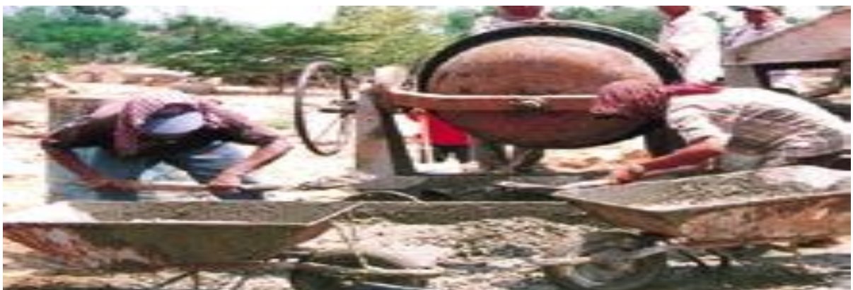
Figure 106: Mechanical mixing
