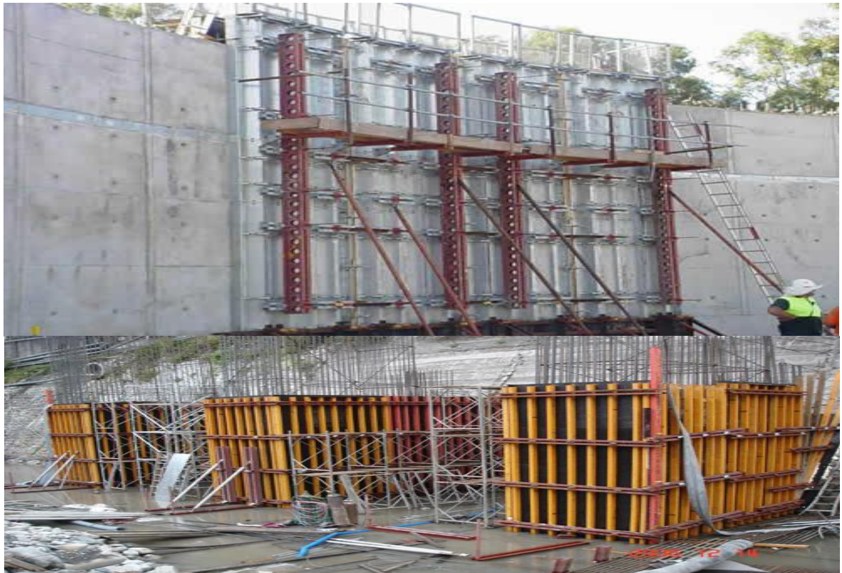
Figure 38: Wall formwork
