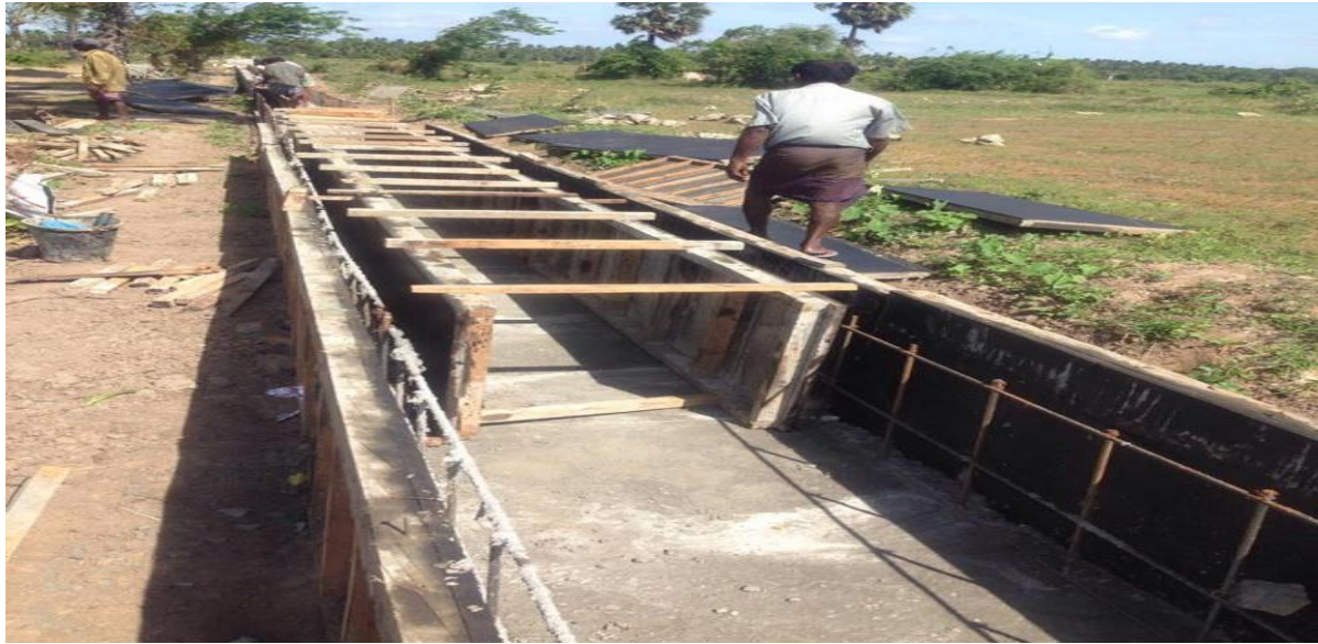
Figure 79: Erecting formwork
