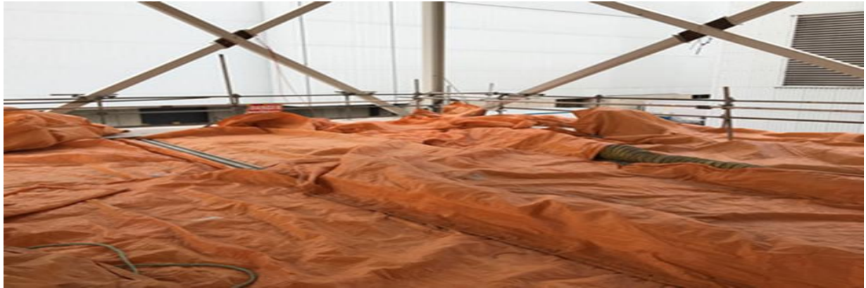
Figure 115: Covering of concrete surface with blanket in cold weather
