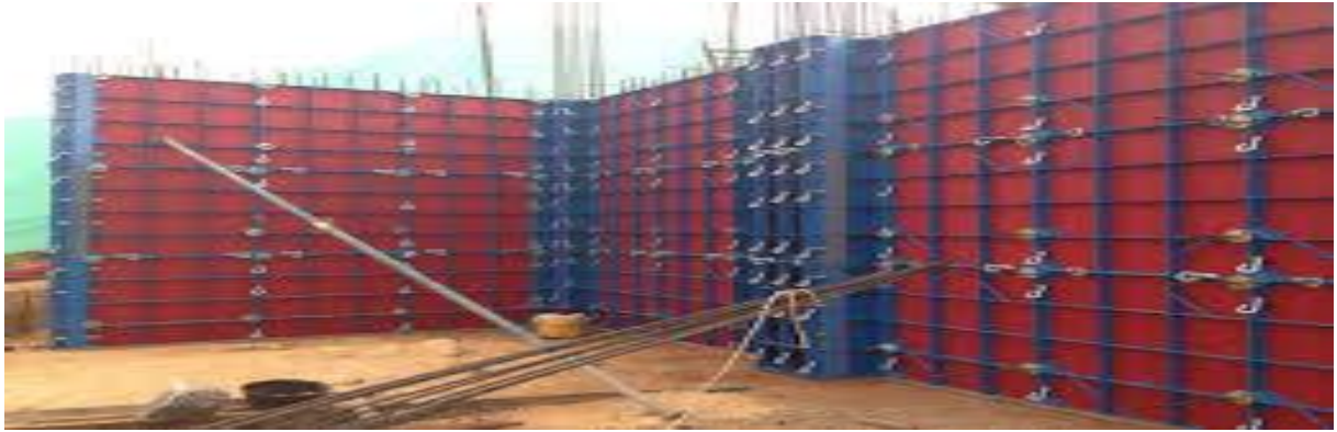
Figure 62: Stiffening rods to panels
