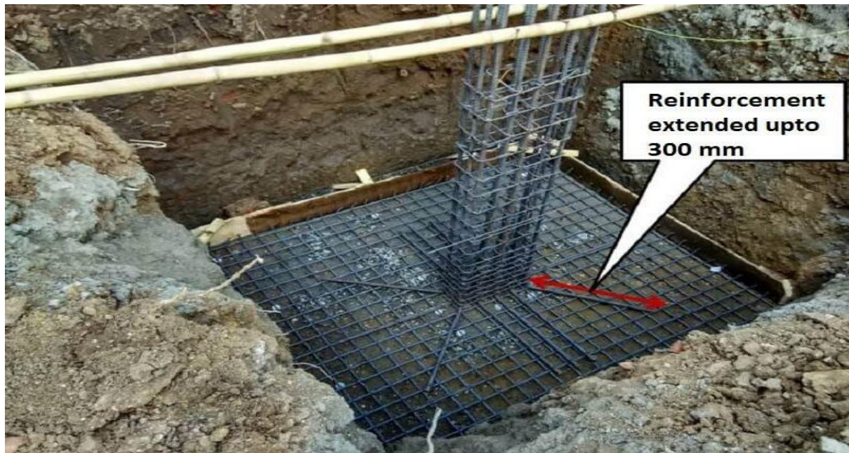
Figure 65: Placing reinforcement in footing
