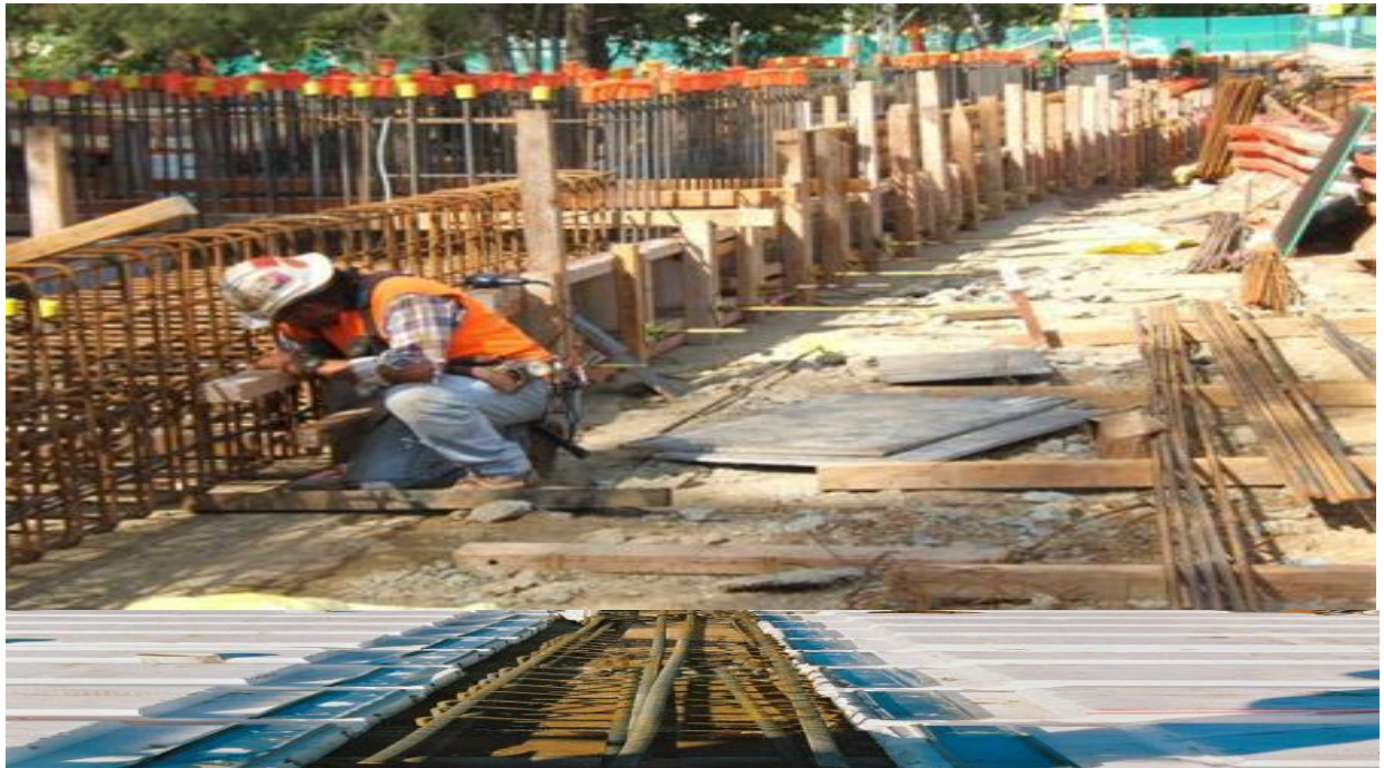
Figure 36: Beam formwork
