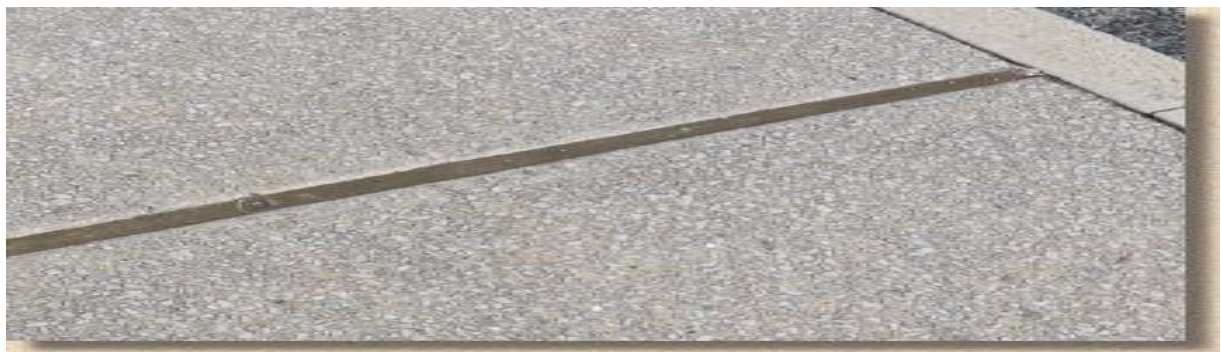
Figure 84: Sealed movement joint
