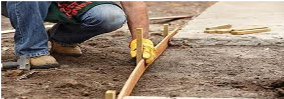
Figure 76: Setting out formwork
