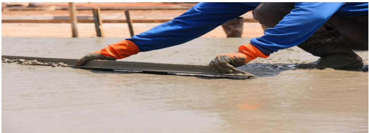
Figure 8: Concrete screening
