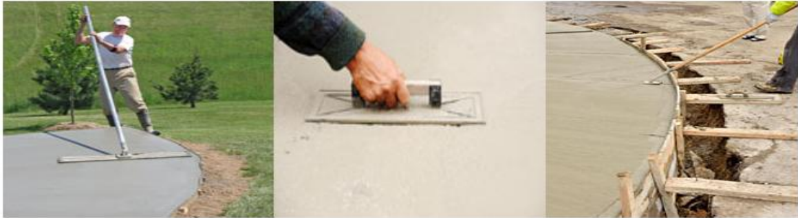
Figure 114: Concrete screening
