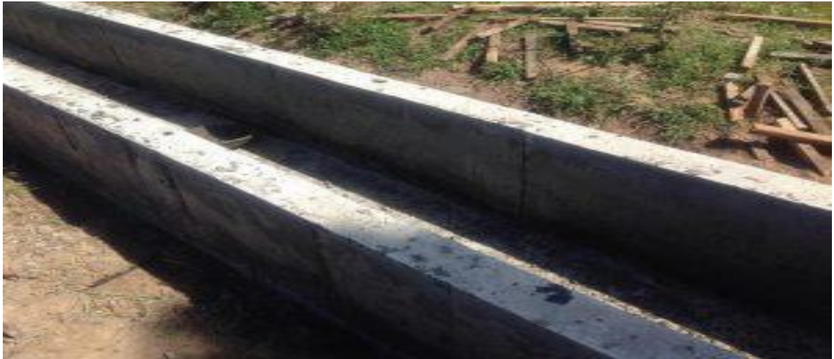
Figure 116: Concrete canal after removing formwork
