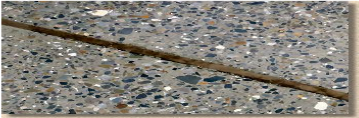
Figure 88: Fiberboard joint in polished concrete slab
