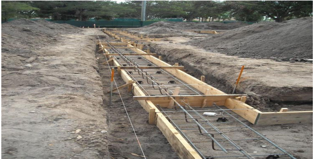
Figure 57: Tying reinforcement bars
