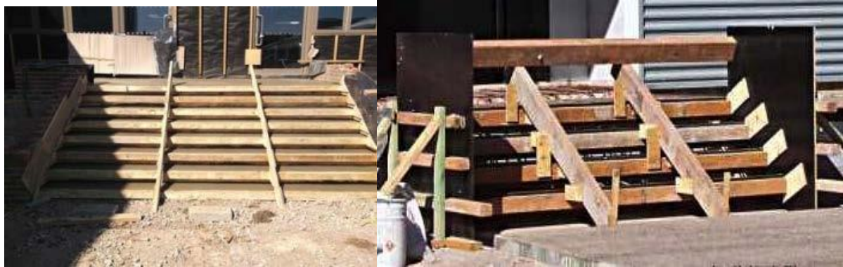
Figure 67: Sole plate of formwork
