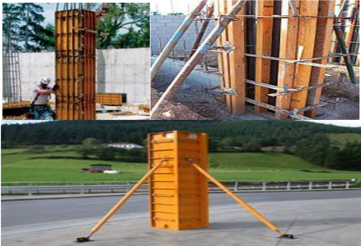
Figure 35: Column formwork
