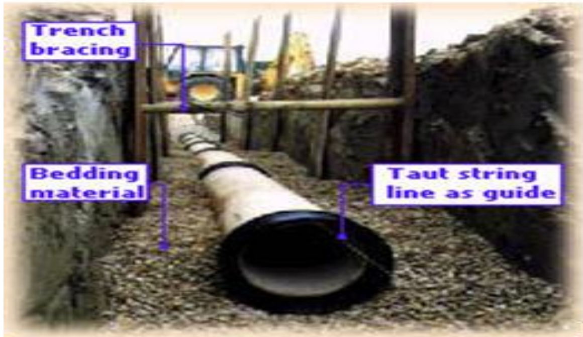
Figure30: Pipe laying
