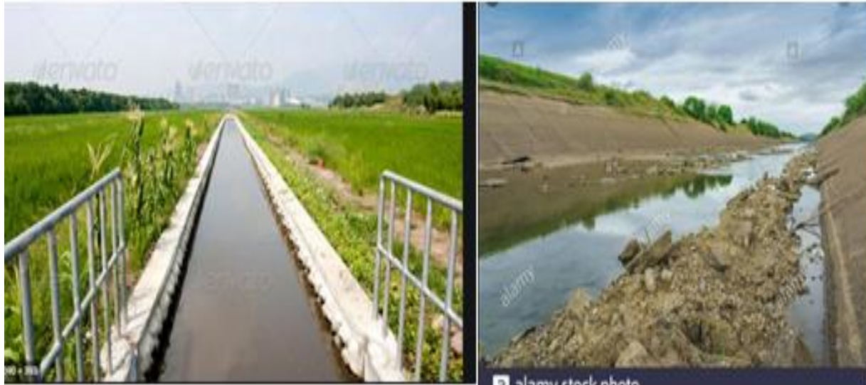
Figure 24 [a]: Operating canal Figure 24 [b]: Silted canal
