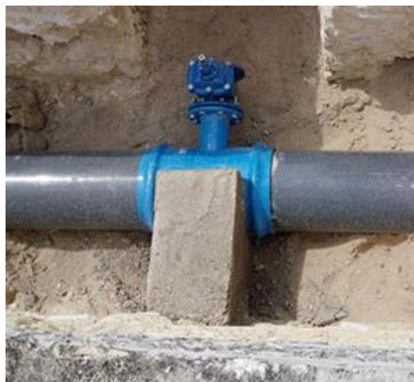
Figure 58. Thrust block
