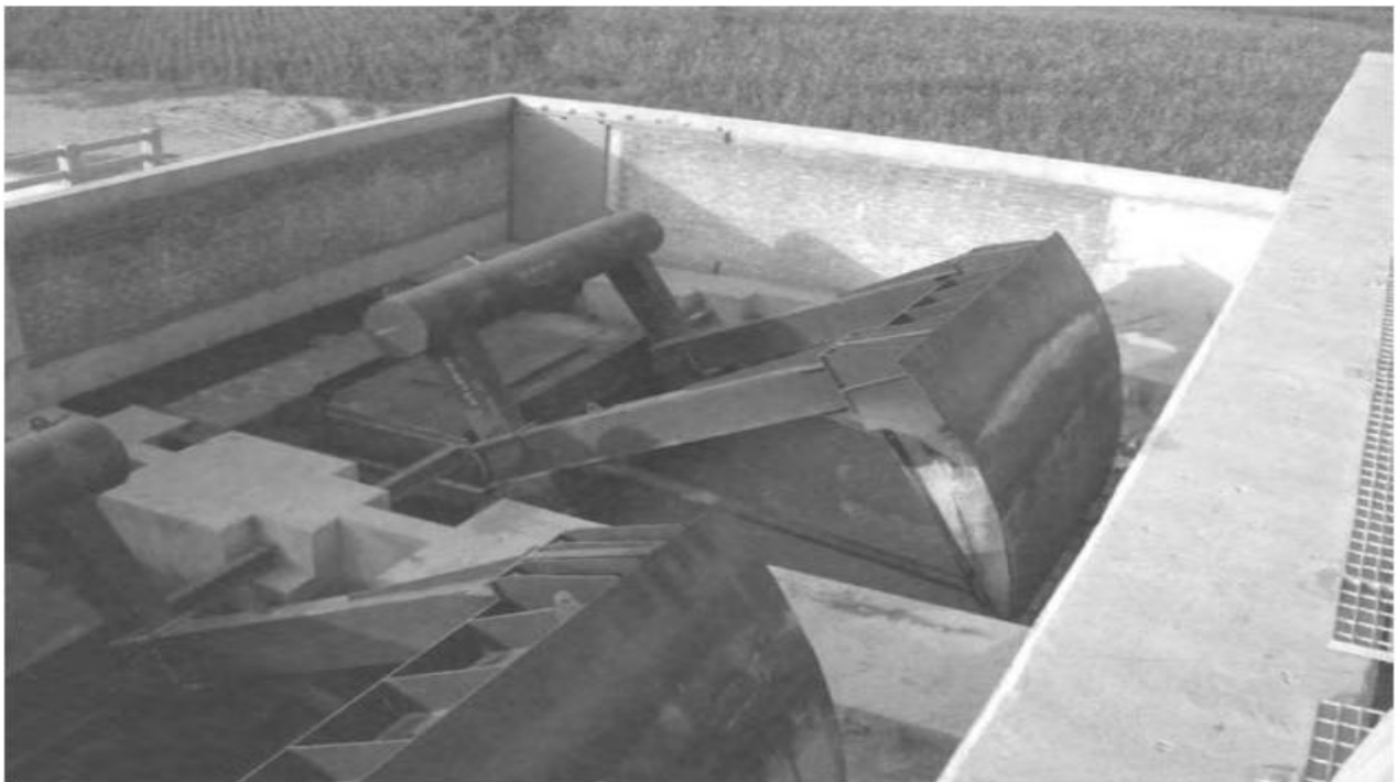
Figure 12: Downstream control gates
