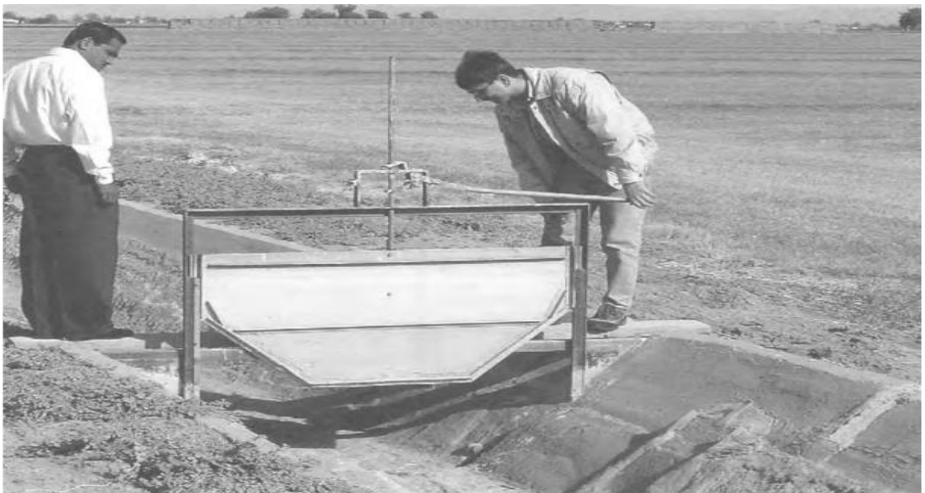
Figure 13: A lever-operated check gate
