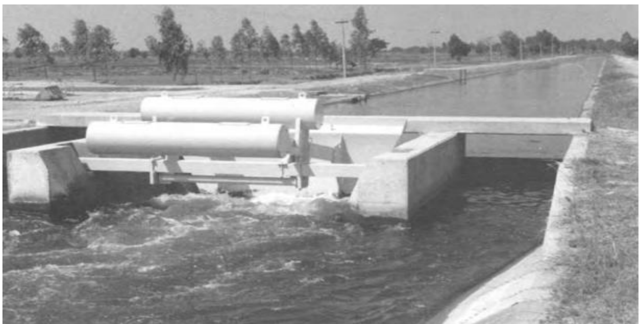
Figure 11: Upstream control by afloat-operated self-regulating gate
