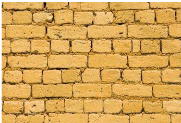
Fig. 1: Brick work in mud
