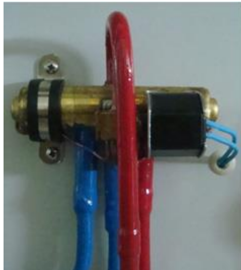
Figure 32. Four-way valve
