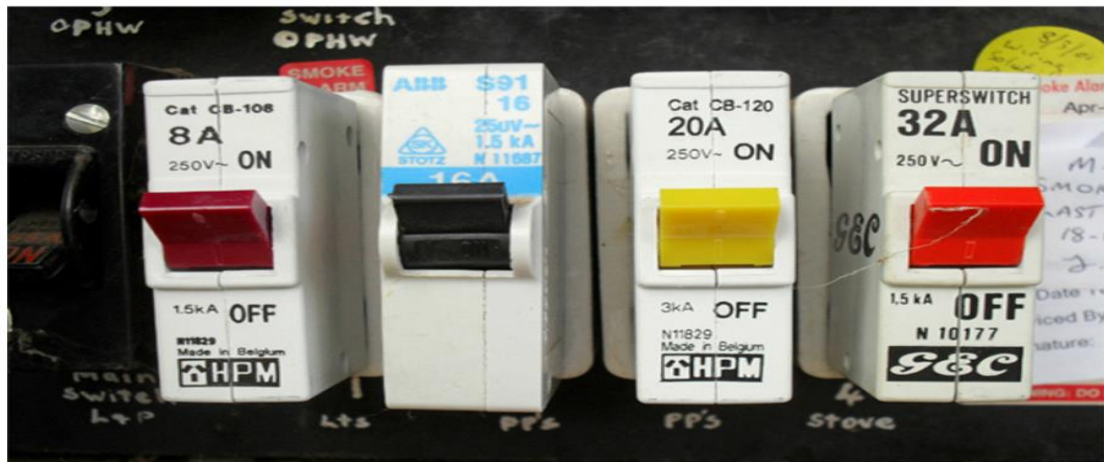
Fig 5.3. Different size and rating of circuit breaker
