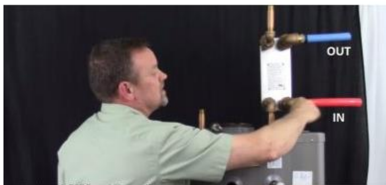
Figure 6. Connecting pipes from the pre-cooler to the inlet
