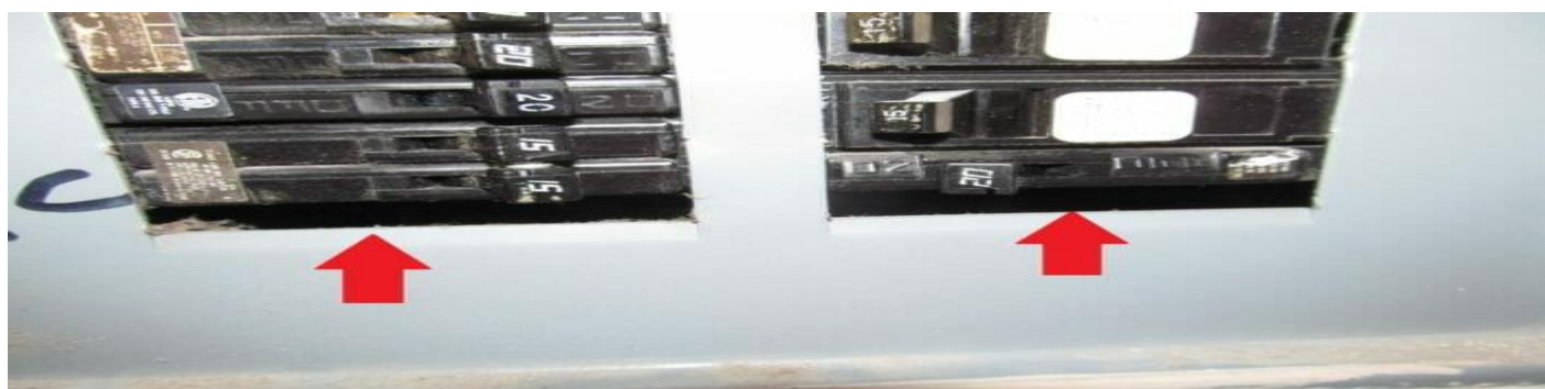
Figure 3-6 Panel missing knockouts
