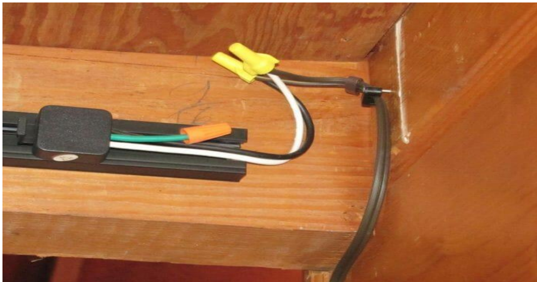
Figure 3-4 Exposed Wiring and Splices
