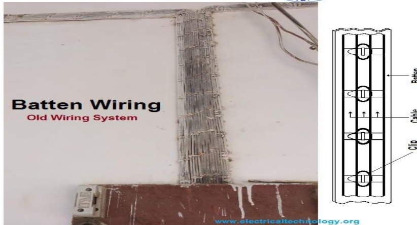
Figure 1-5 batten wiring
