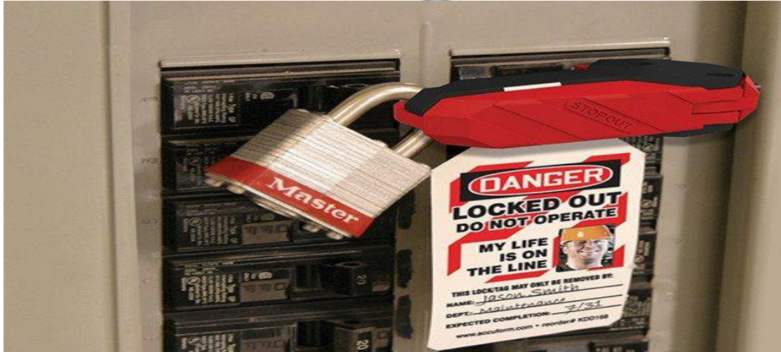
Figure 1-6 Circuit breaker lockout tag (photo credit: lockoutstore.com)
