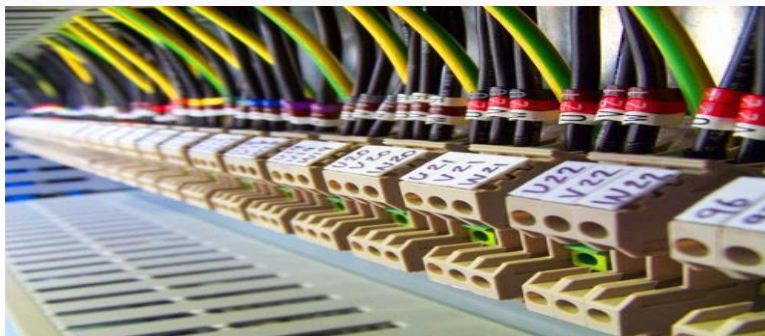
Figure1-3 Identification of conductors
