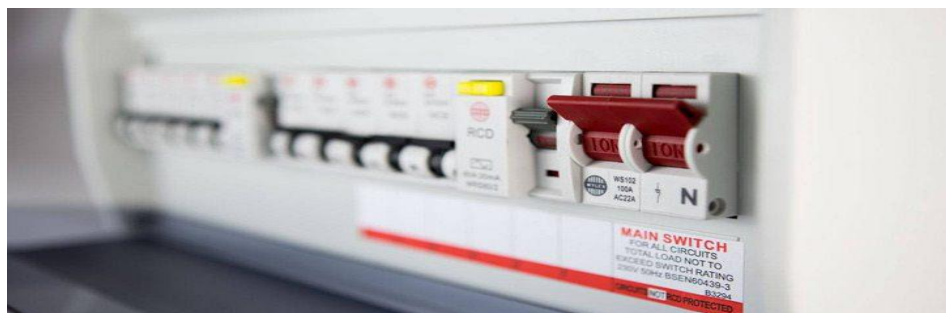
Figure 1-5 Protective devices – Miniature circuit breakers (photo credit: electricalsafetycertificate.co.uk )
