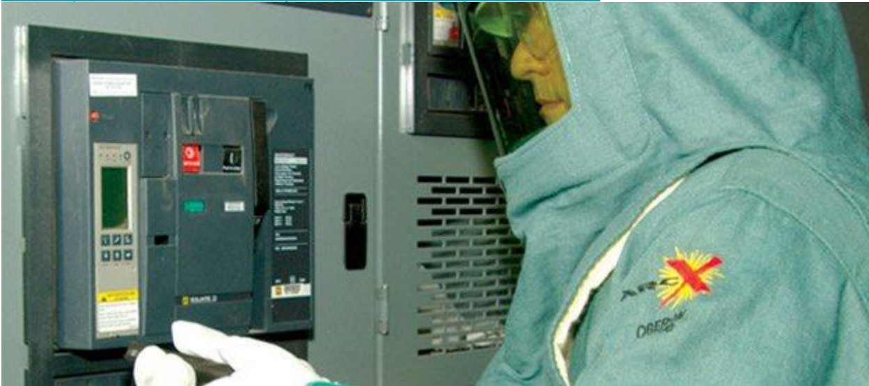
Fig. 2. Disconnect the power source
