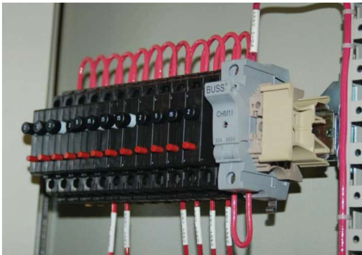
fig 33 Fitting over-voltage protection devices to all cable pairs
