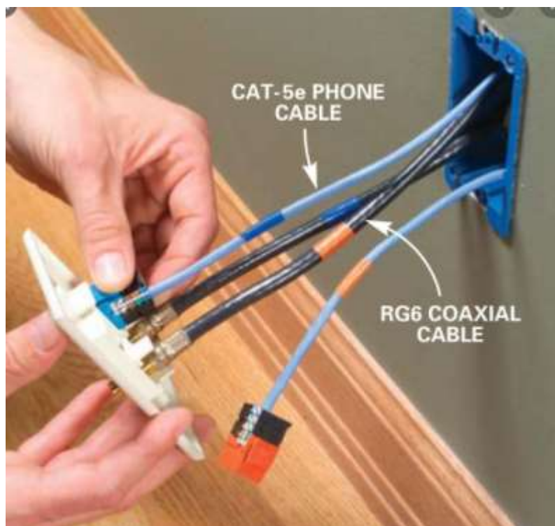
Fig 28.RG6 coaxial cable
