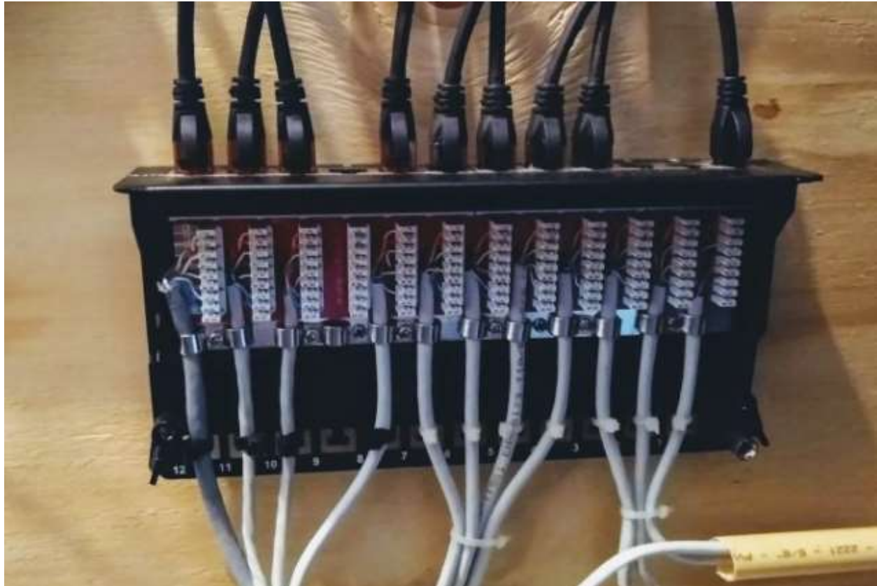
fig 30. Placing and securing cable
