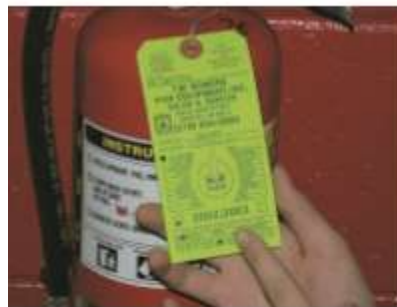
FIGURE-----Someone in the shop must inspect the dates on all fire extinguishers. They must be recharged at periodic intervals.
