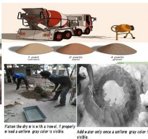
Fig.2.4 Open hill and add water ready for mix
