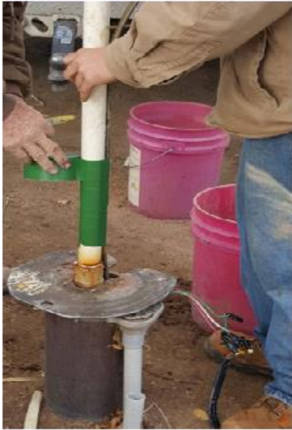
Installing new submersible pump, securing wire and connecting pump wiring.
