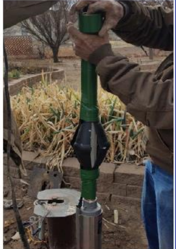
Installing new submersible pump, securing wire and connecting pump wiring.
