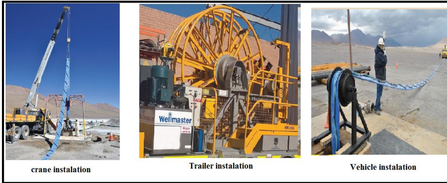
Figure: Dewatering installation methods
