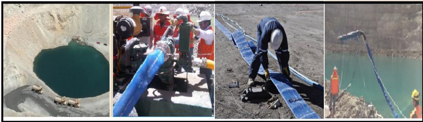
Figure: Dewatering hose installation
