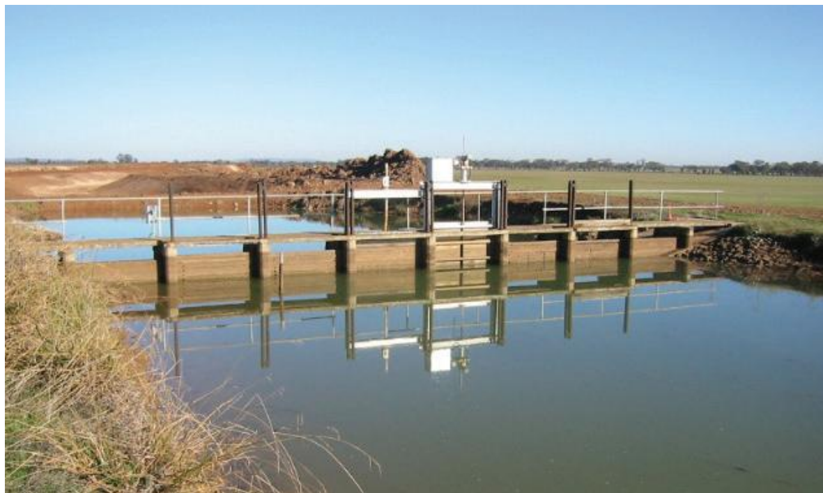
Figure 1: Overshot channel regulator
