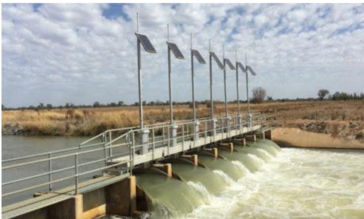
c. Multibay flume gate regulator
