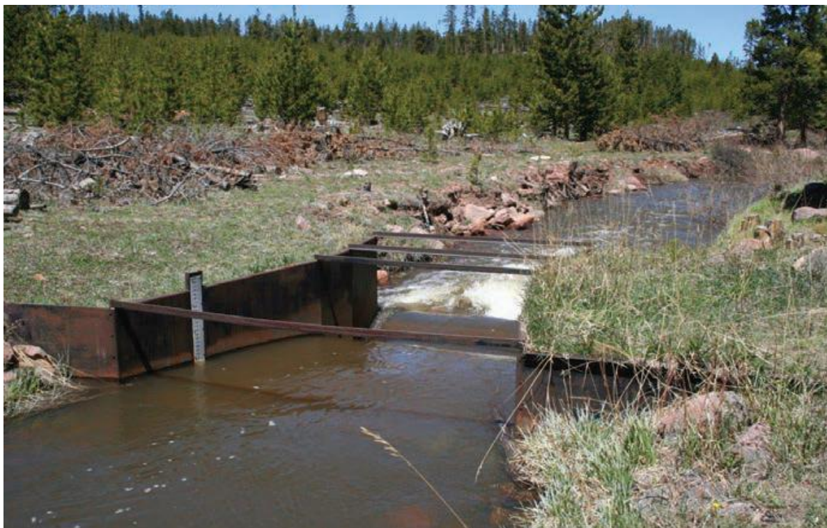
Figure 44: Parshall flume in action
