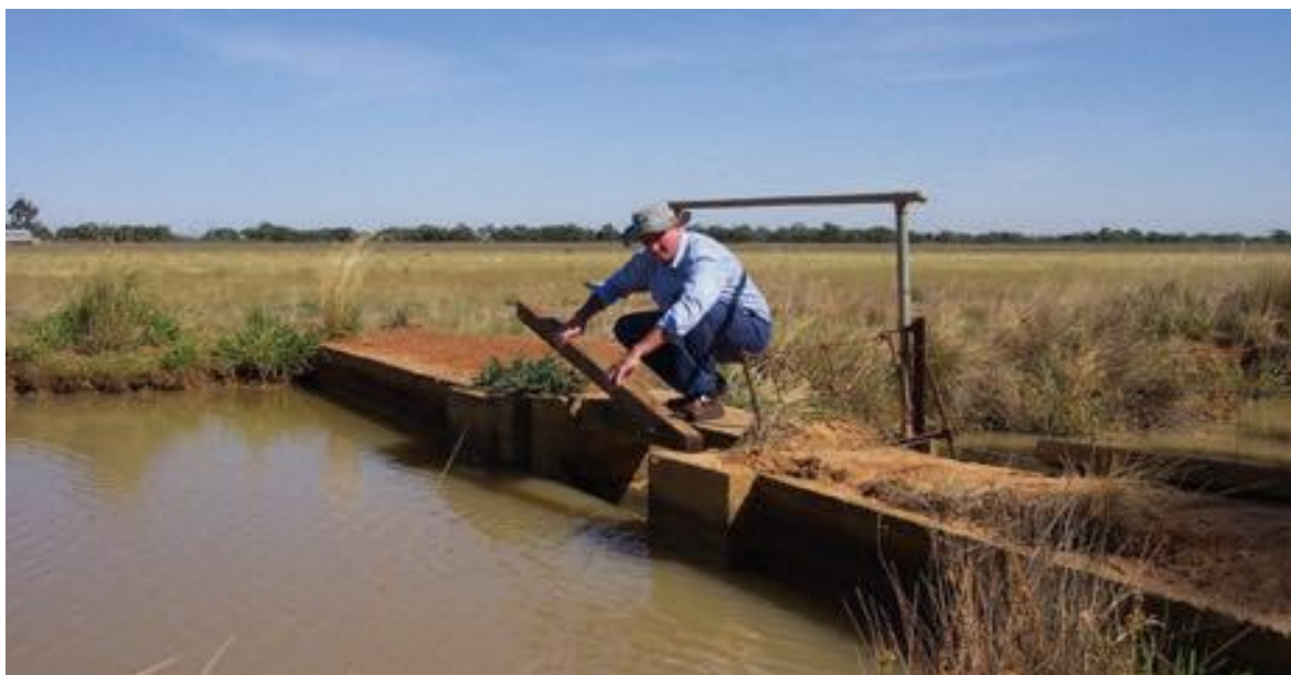
Figure 2: Manual drop bar adjustment of water level at tail regulator
