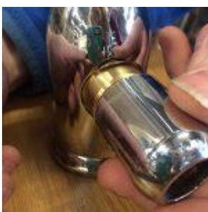
Fig :6.7 Twisting off Shroud covering the valve (or remove if there is a grub screw underneath that you will loosen with Allen Key).
