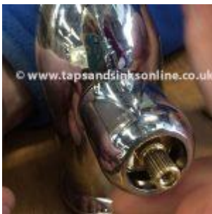
Fig: 6.6 Shroud still covering the Valve which also needs to be removed.
