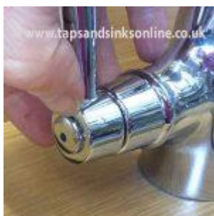
Fig: 6.4 Removing Indicator from Tap Handle to access screw underneath.
