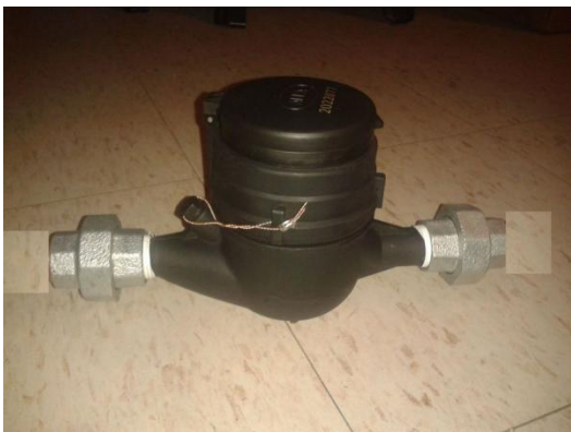
Fig :-6.12 Water meter part
