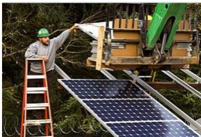
Figure 1: Installing solar panels
