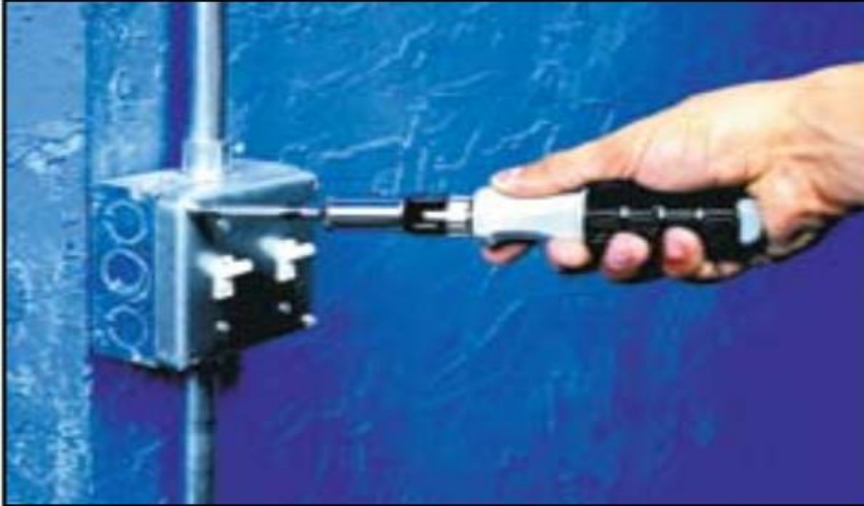
Figure 7.7 Metal electrical boxes grounded to prevent shocks
