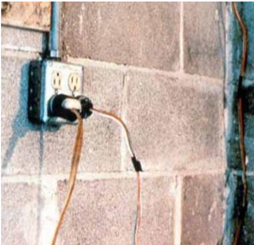
Figure 7.2 damaged extension cords & tools Figure 7.3 damaged extension cords & tools
