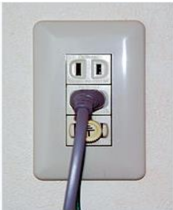
Figure 4.1 Power cord, with plug at end, plugged into an outlet with ground post
