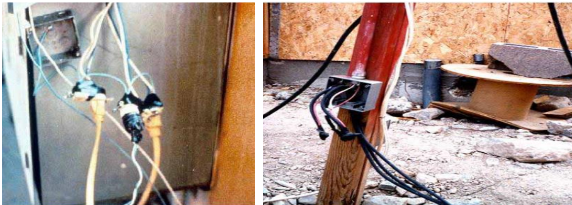
Figure 7.1 exposed and unsafe electric cord assemblies
