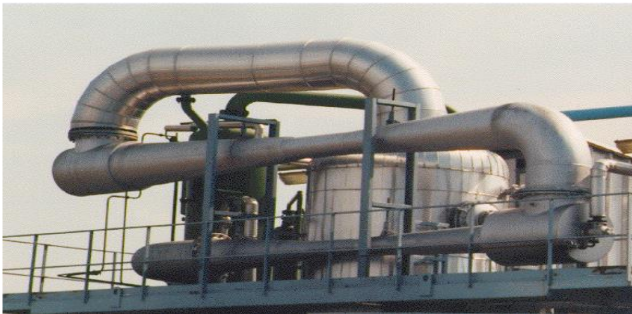
Figure 5 multi-stage ejector vacuum systems
