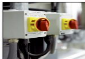
Motor disconnect
