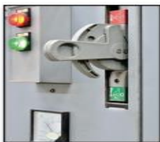
Main disconnect switch
