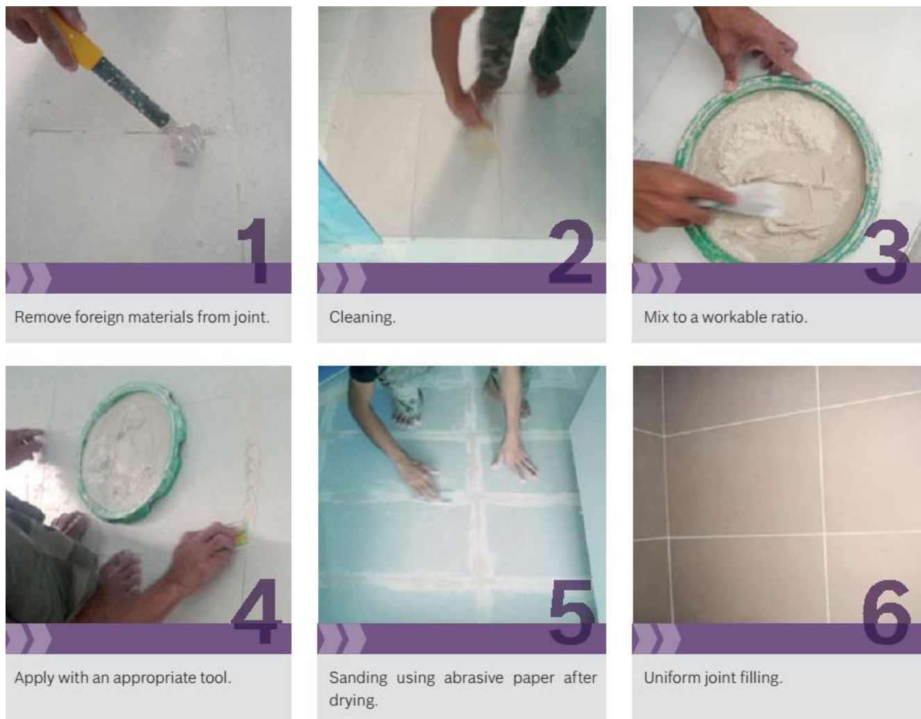
Fig. 4 – Application of grout in ceramic tiling.
