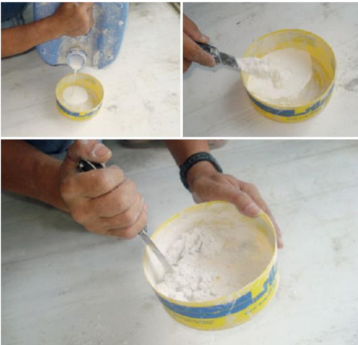
Fig. 3 – Adding liquid polymeric additives to cement grout enhances its performance.
