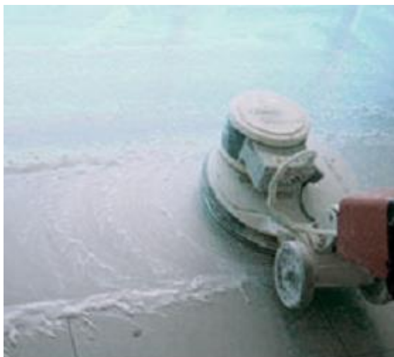
Fig. 5 – Wet polishing on a marble floor.
