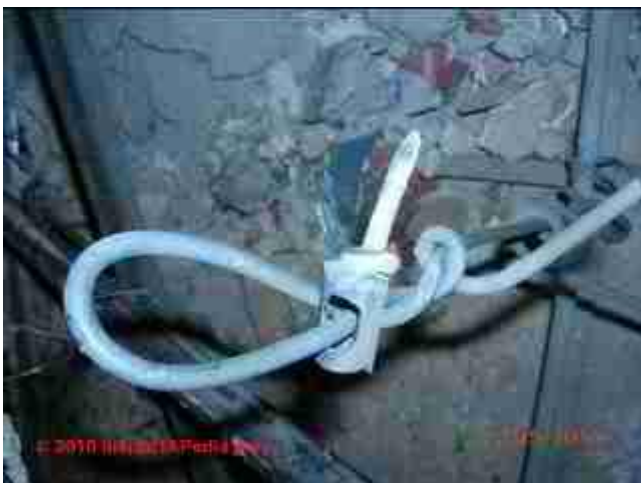
Figure 5.3 Metal Lath Plaster Ceiling Collapse Cause
