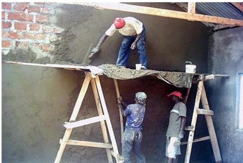
Fig 1.2: Plastering Work
