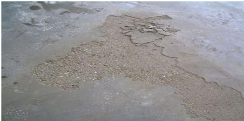
Fig1.4 Delamination
