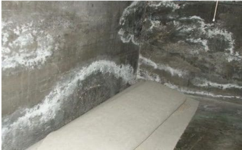
Fig1.7 Efflorescence
