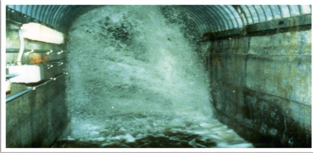
Fig2.1 High-volume water leaks can be repaired using Epoxy resins
