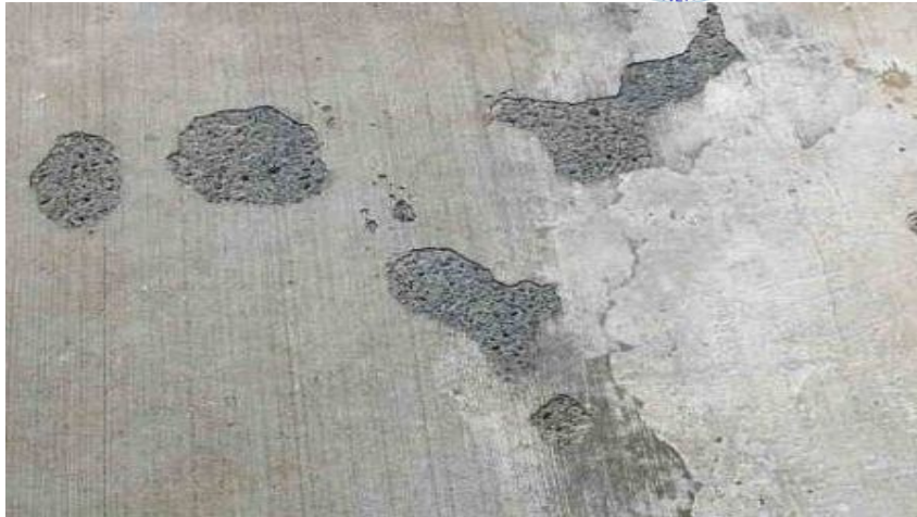
Fig1.3 concrete blistering
