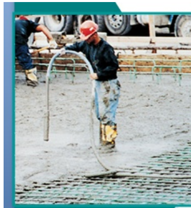
Fig3.6. Placing Concrete in a Sloping Lift
