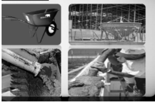
Fig3.4 Transporting of concrete
