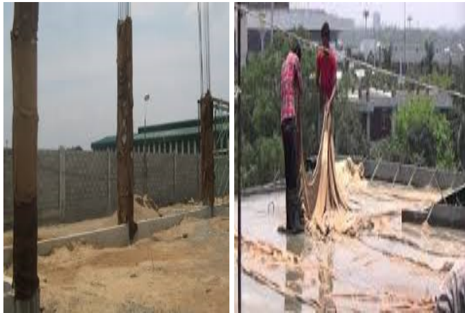
Fig3.3 covering concrete
