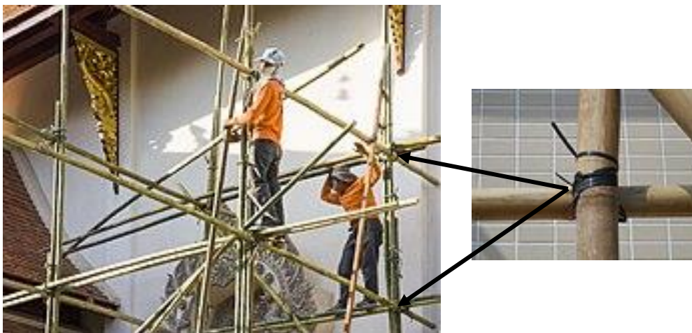
Figure 6.2 Bamboo Scaffolding
