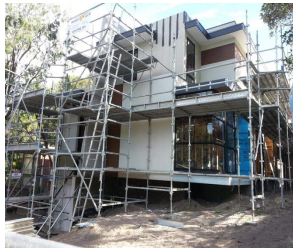
Figure 1.1 Scaffolding is used
