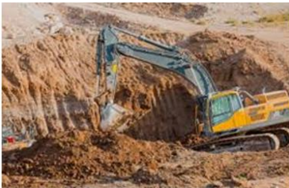
Fig-7 Bulk excavation
