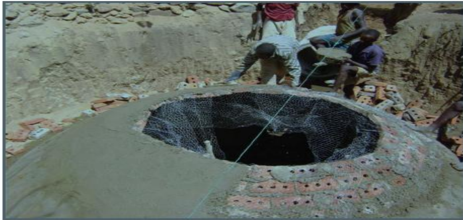
Figure 19.6:- An anaerobic digester under construction
