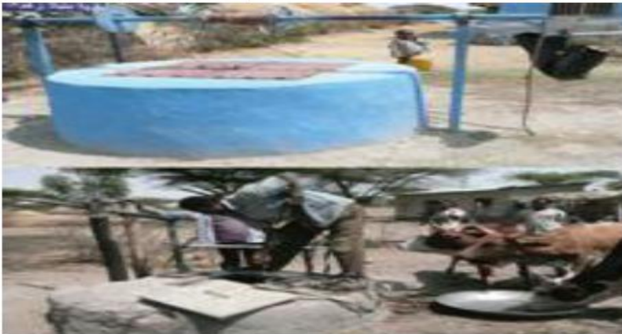
Figure 9.4: Two wells with concrete protection.
