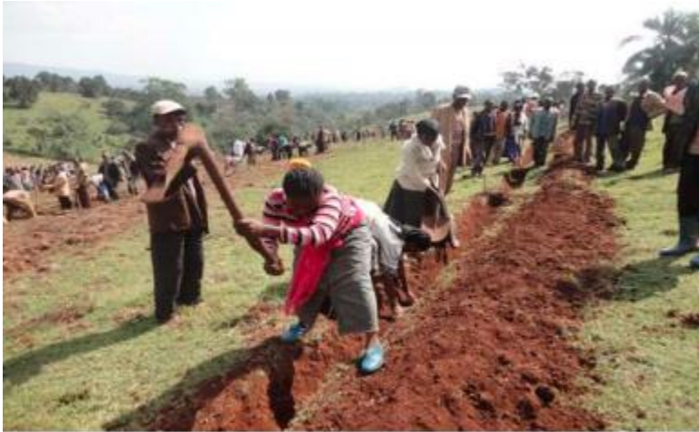
Figure: 5.6.1 Soil and water conservation structure under construction.
