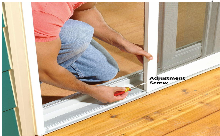
Figure 4 adjustment screw
