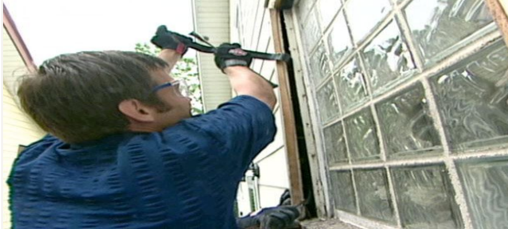
Figure 7 removing frame
