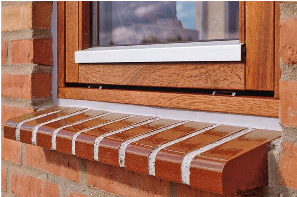
Figure 5 window sill bricks
