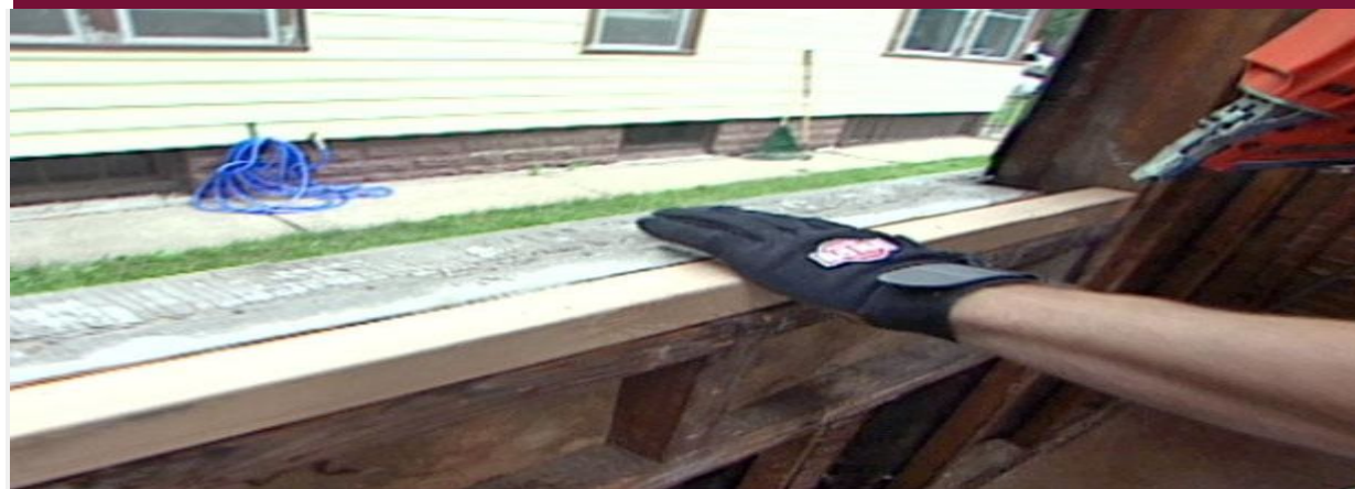
Figure 10 form the new sill
