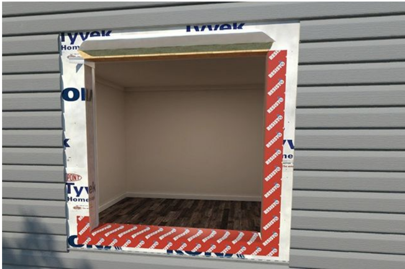
Figure 12 prepare the opening
