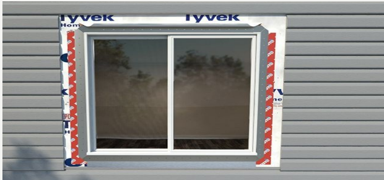
Figure 13 window installation
