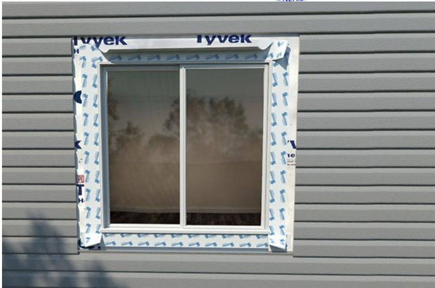
Figure 15 waterproof the window
