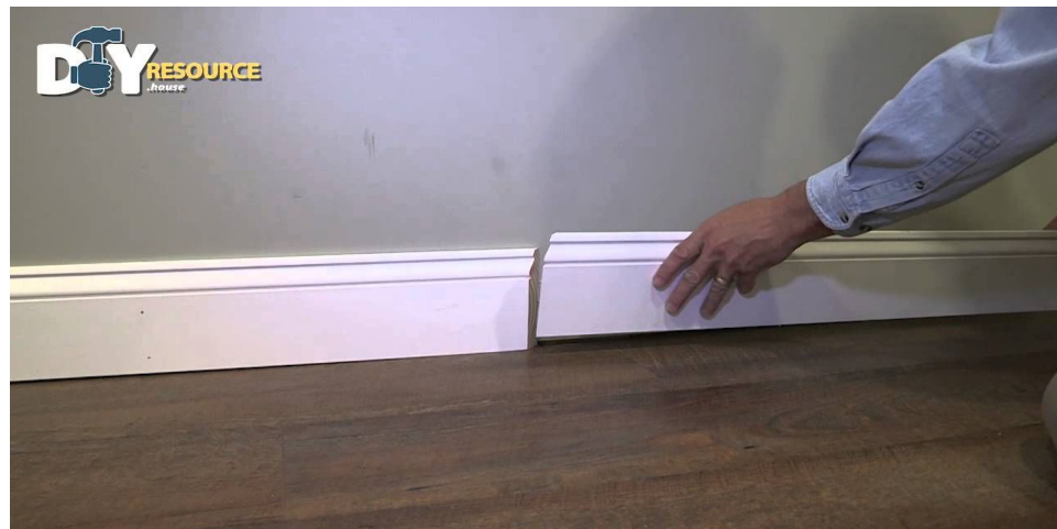
Figure 13 installation of scarf joints
