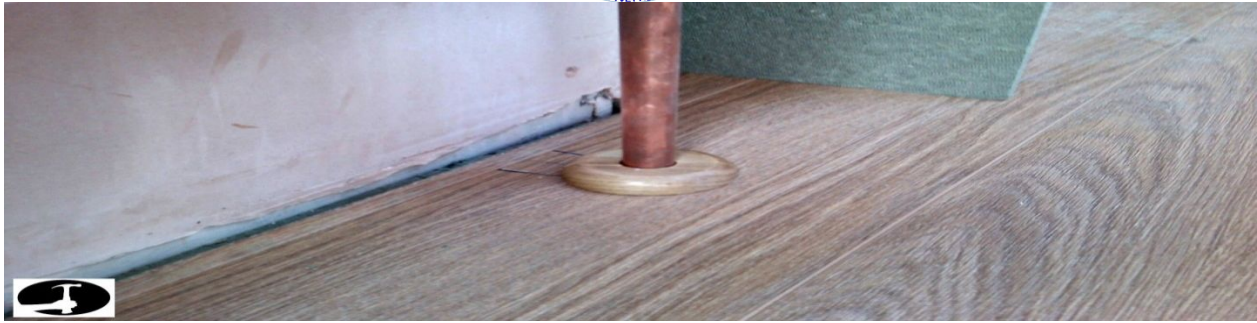
Figure 10 drill hole of the pipe
