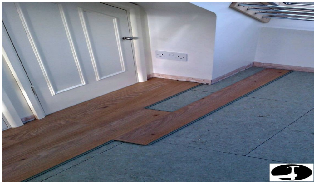
Figure 8 setting out boards
