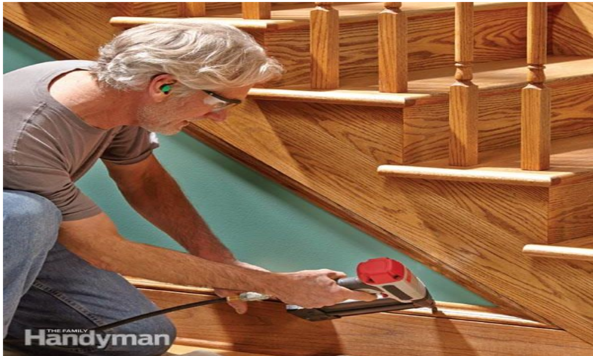
Figure 9 fixing paneling
