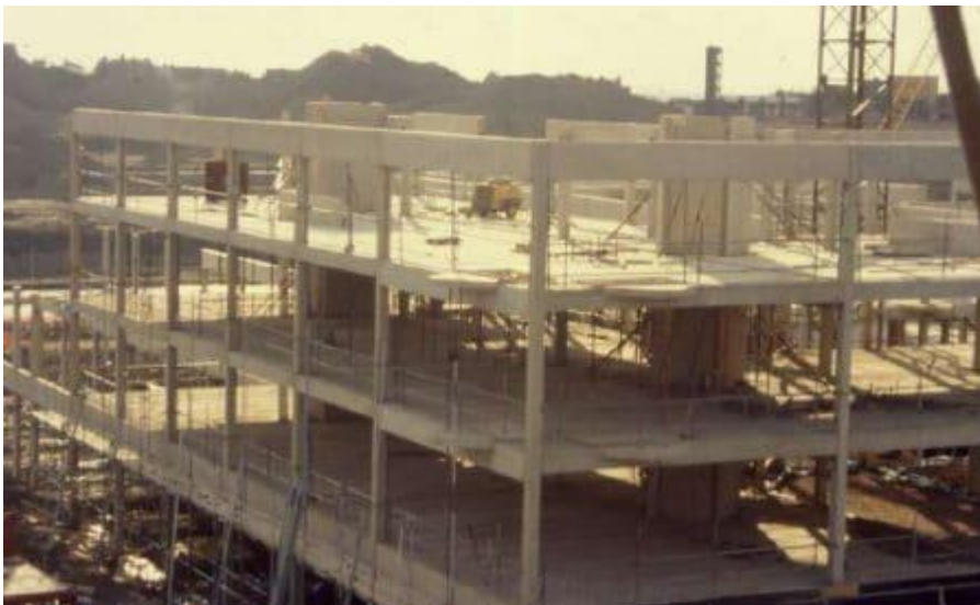
Fig. 4.3: Precast Concrete Frame Structure erected within four weeks
