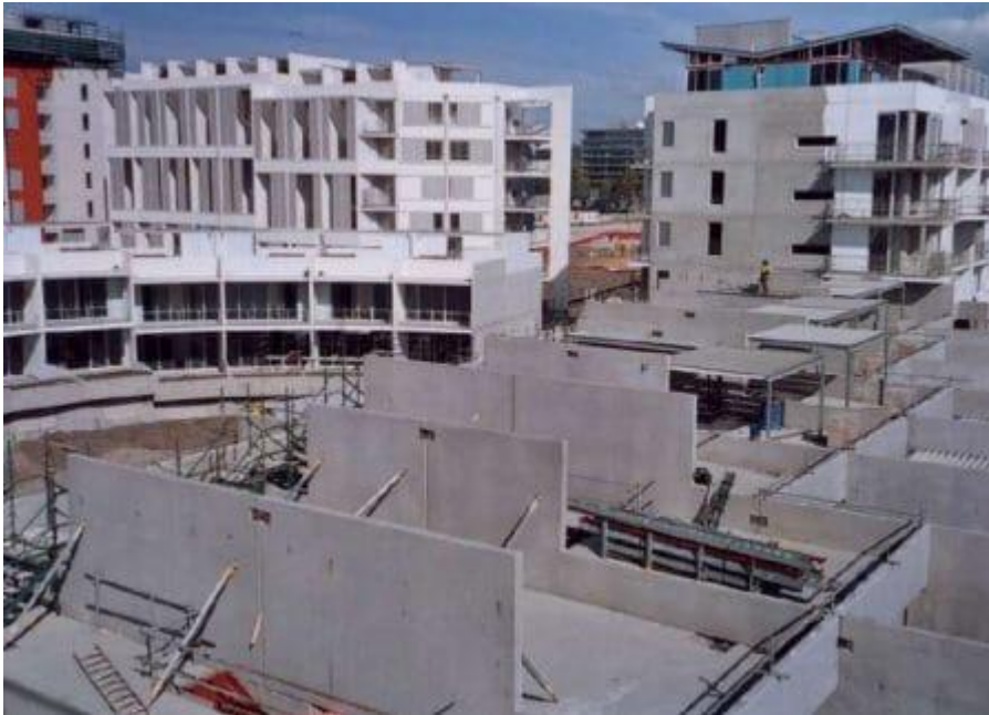
Fig. 4.2: Large Panel Precast Concrete System Construction
