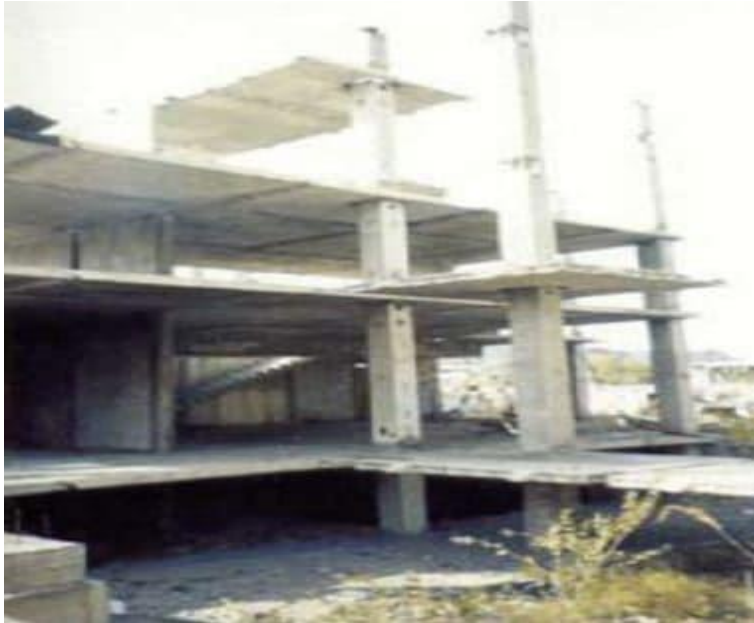
Fig. 4.4: Precast Column-slab System with Shear Walls
